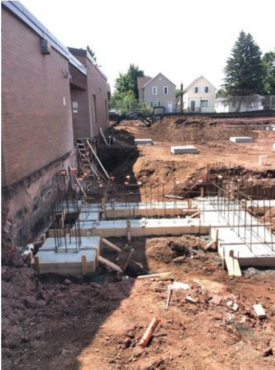
Footings and foundation ongoing at Cafetorium Addition
