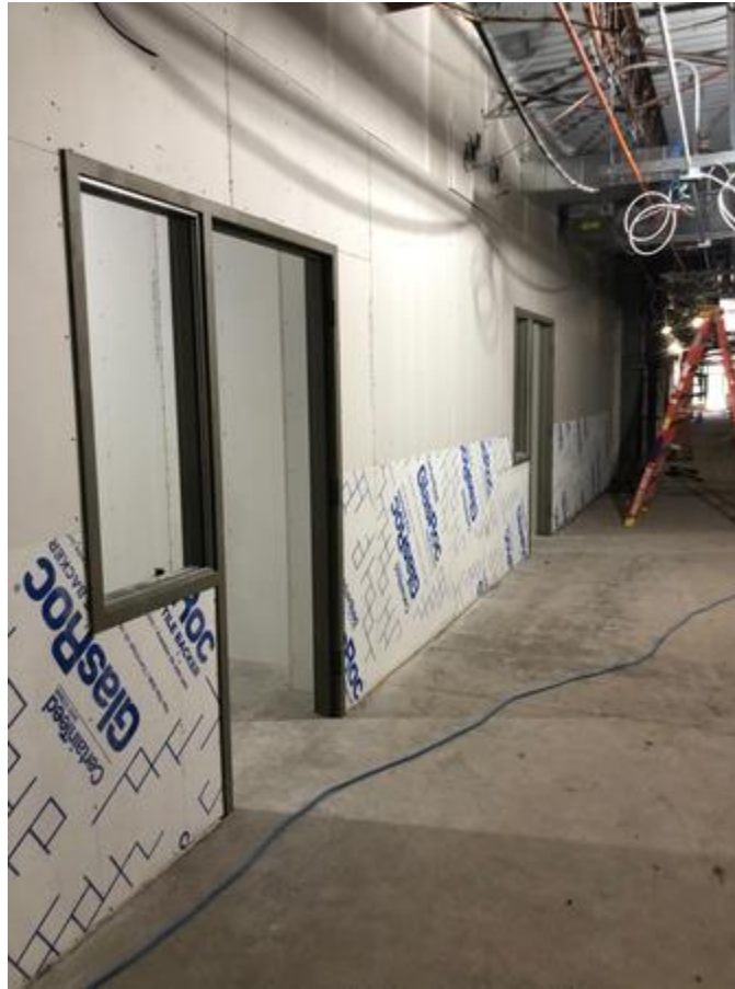
Sheetrock ongoing throughout.
