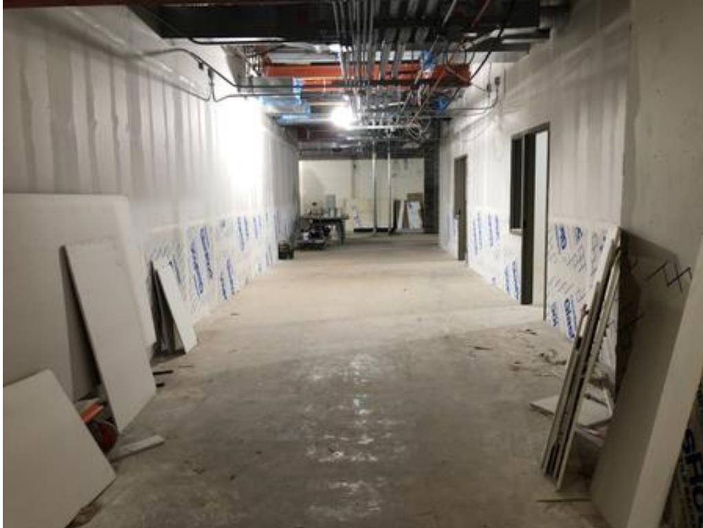
Sheetrock finishing in areas. Mud and tape ongoing. Painting to follow
