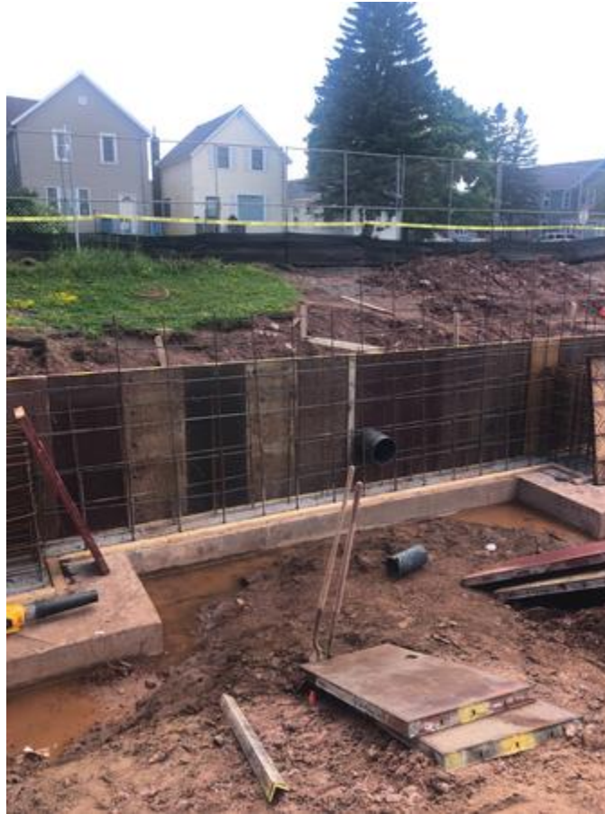
Footings and foundations ongoing at Cafetorium Addition
