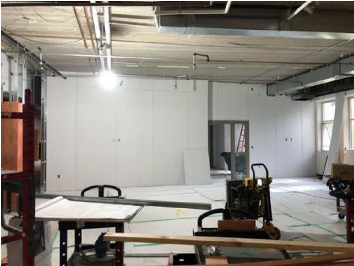
Sheetrock walls finishing up.
