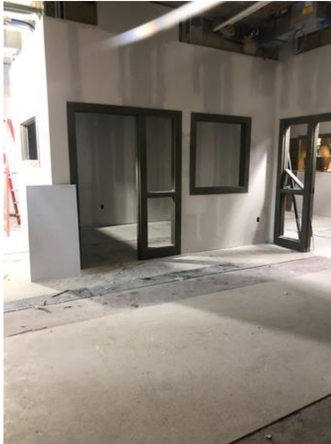
Sheetrock walls finishing up.
