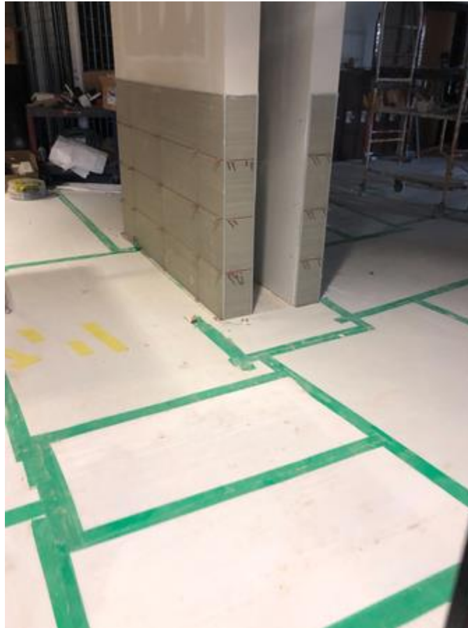
Tile install ongoing
