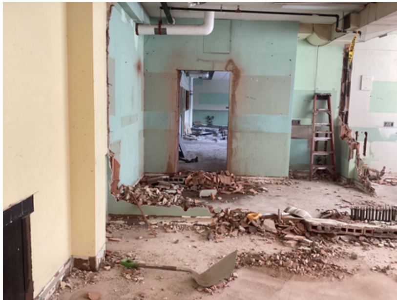
Science Rooms Demolition
