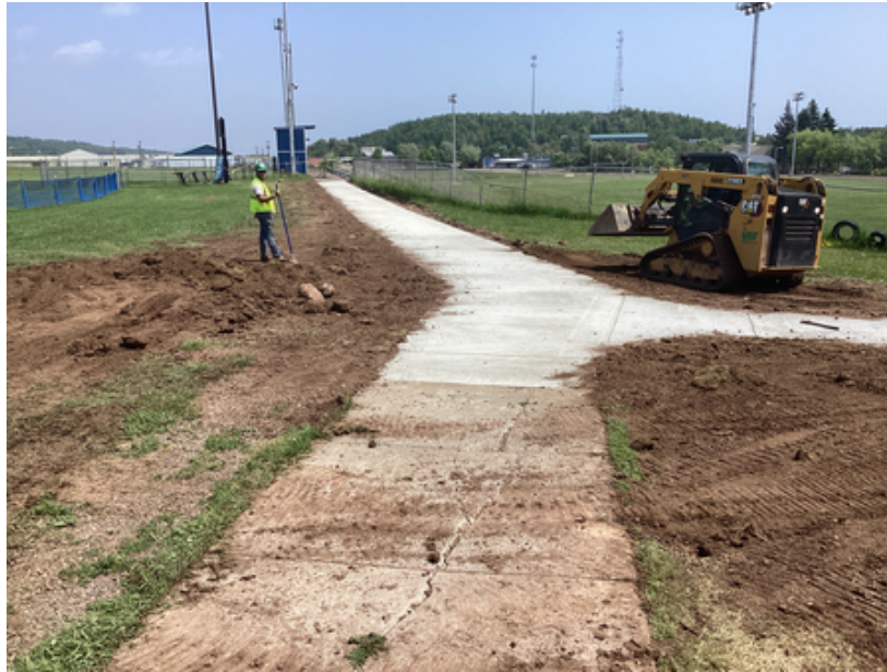
Exterior sidewalks backfilled.
