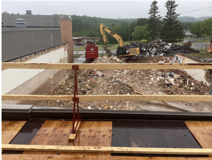
Music Suite Demolition
