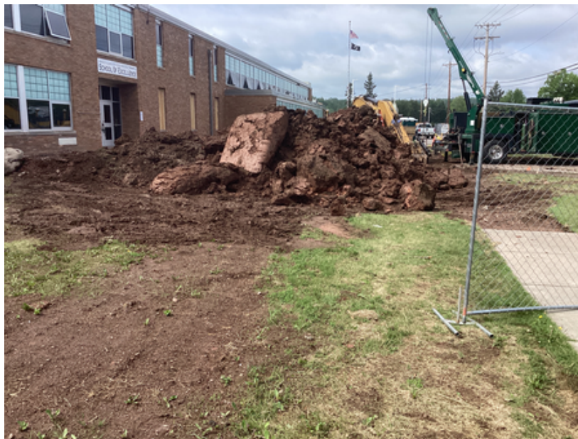
Continued excavation for Main Entrance addition
