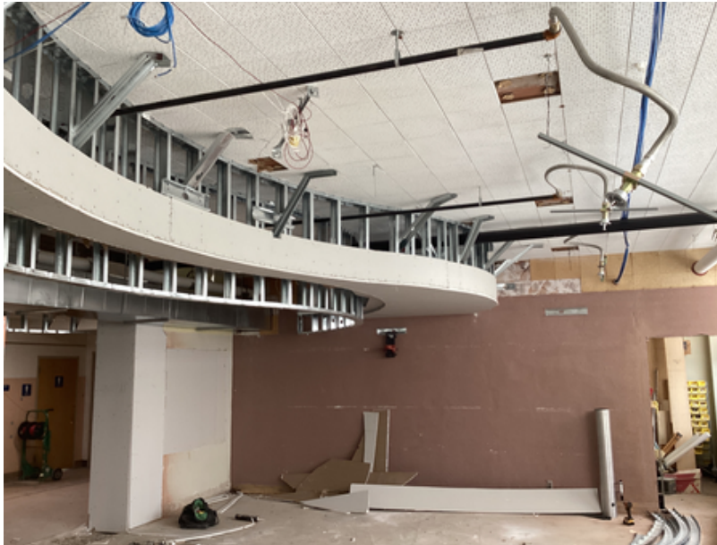
New Flex Room Soffit Framing
