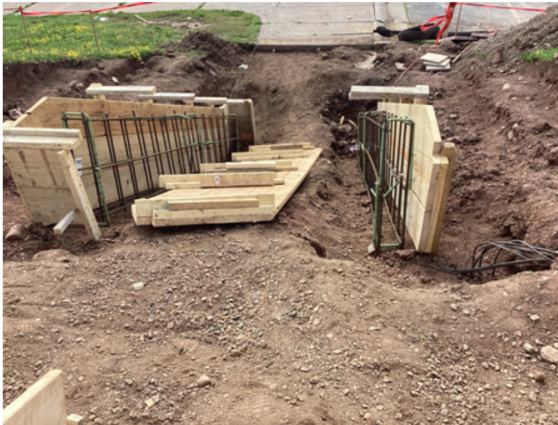
Forming of concrete stair replacement
