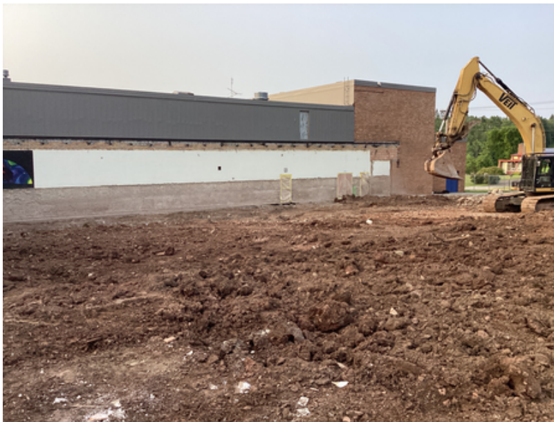
Music Suite Demolition
