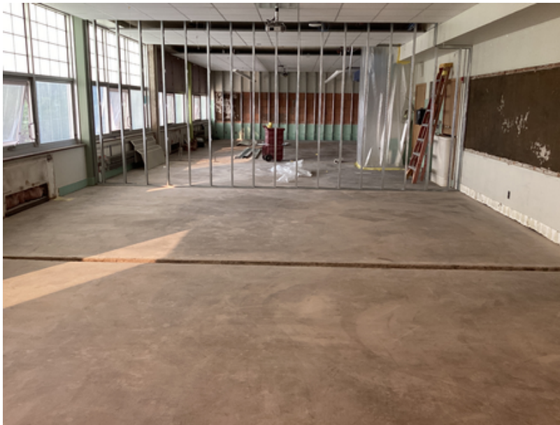
Classroom Wall Framing
