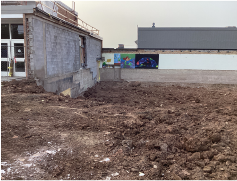
Music Suite Demolition
