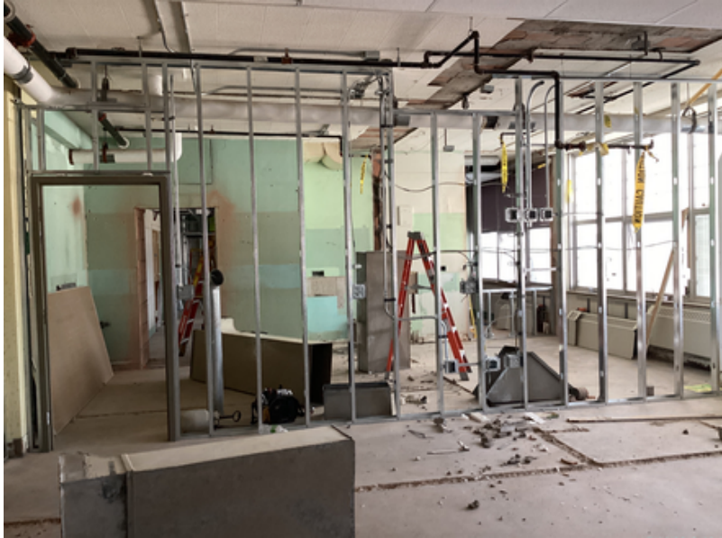
Science Rooms Wall Framing
