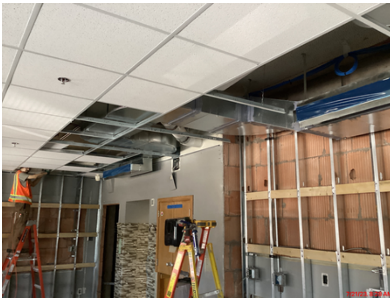
Classroom, electrical, mechanical rough in and wall framing
