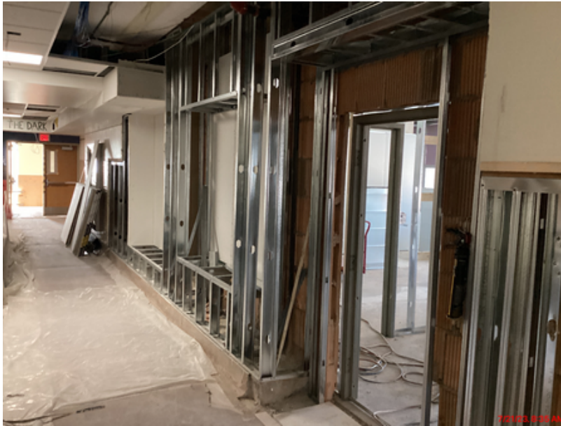
Hallway outside of Science Classroom wall and display framing
