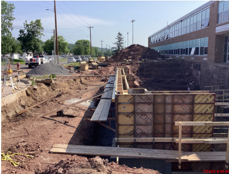
Forms, footings, and foundations poured for the new main entrance addition.
