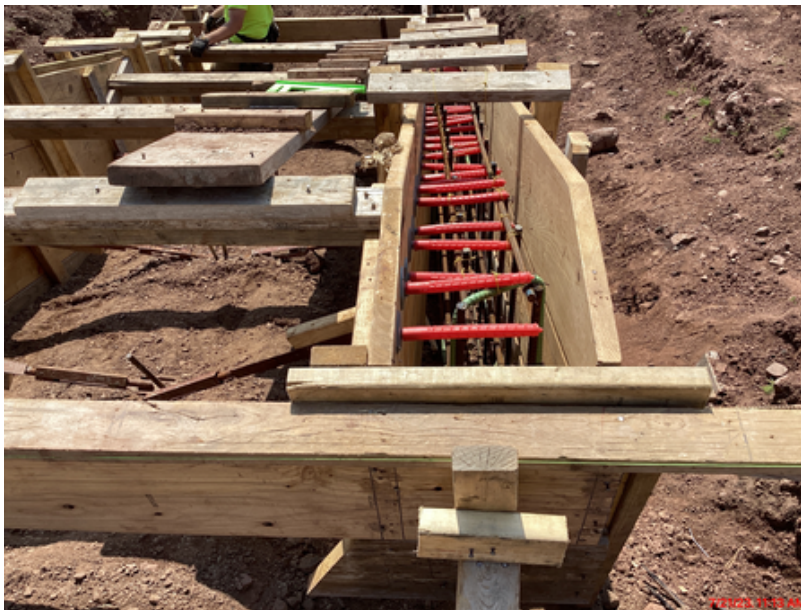
Forming of concrete stair replacement
