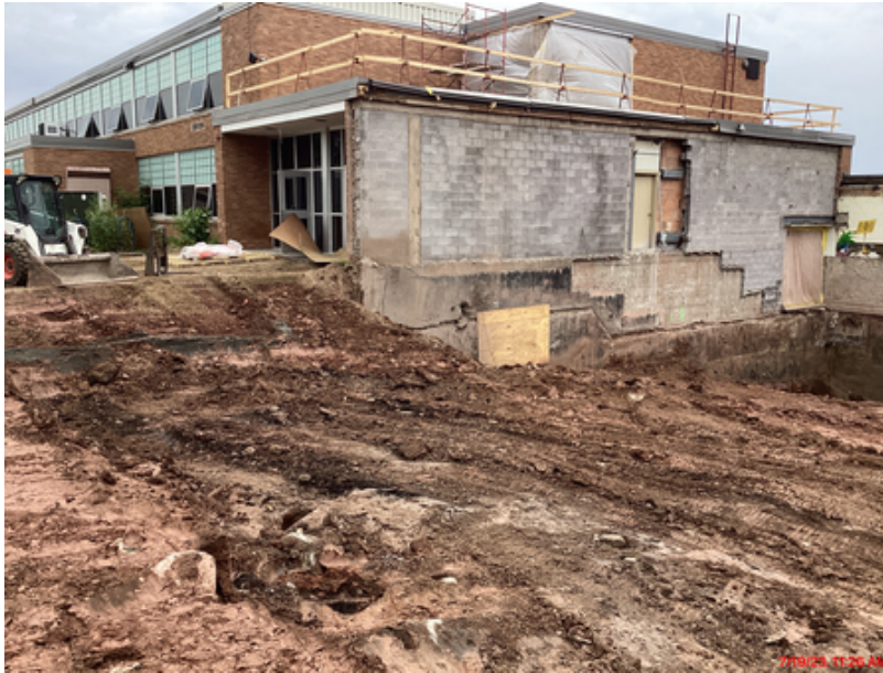
Excavation for footings and foundations for the new music suite addition
