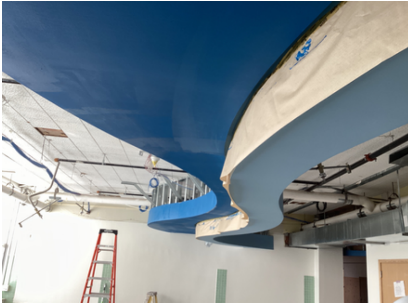
Painting soffits in new flex space
