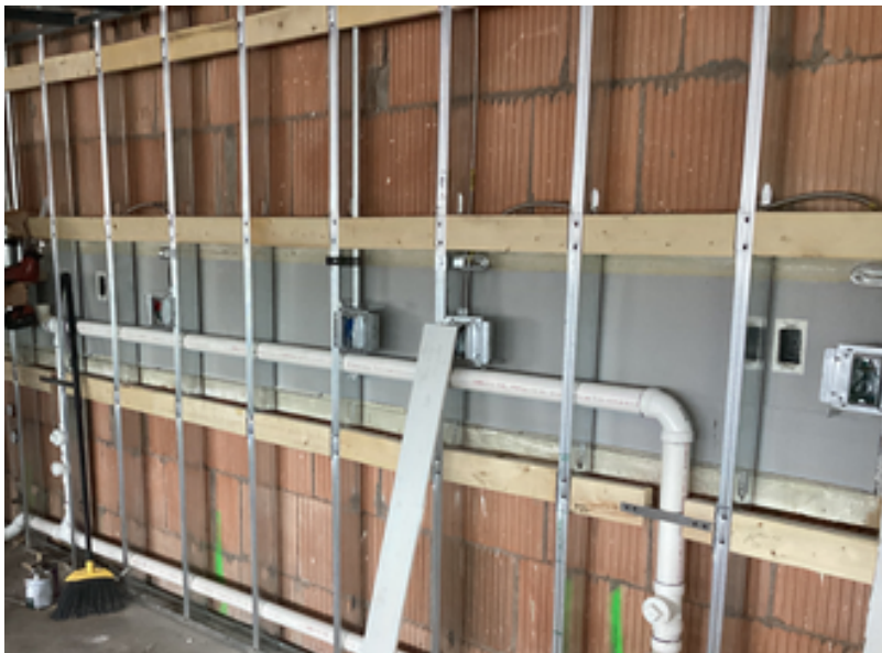
Science Classrooms plumbing and electrical rough ins.
