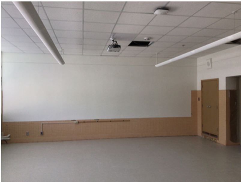
Classroom painting and floor installation
