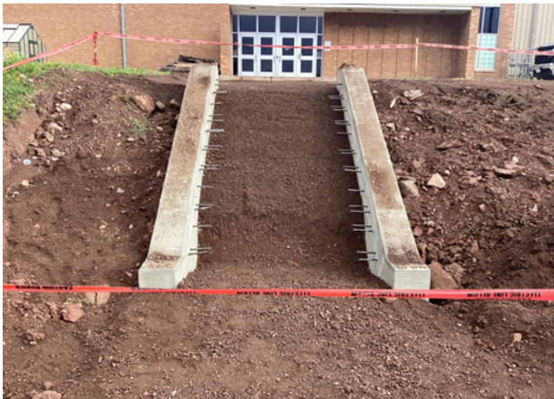
New stairwell walls poured.
