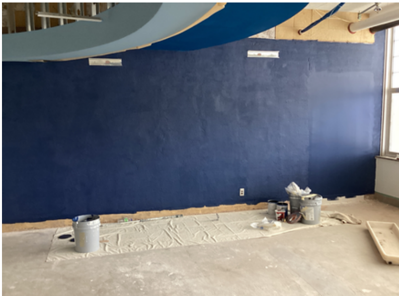
Painting walls in new flex space
