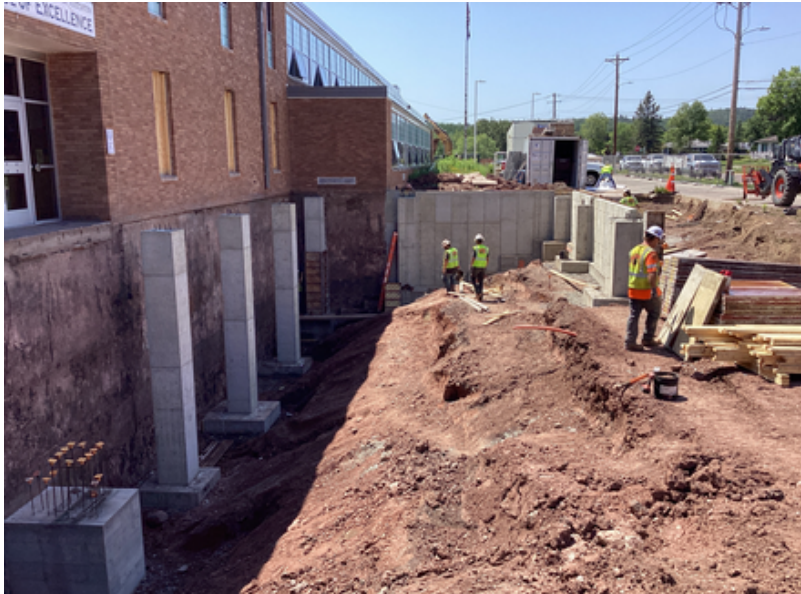
Footings and foundations poured for main entrance addition.
