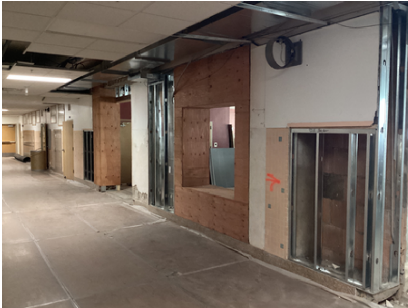
Outside of Media Center Wall and Display Case Framing
