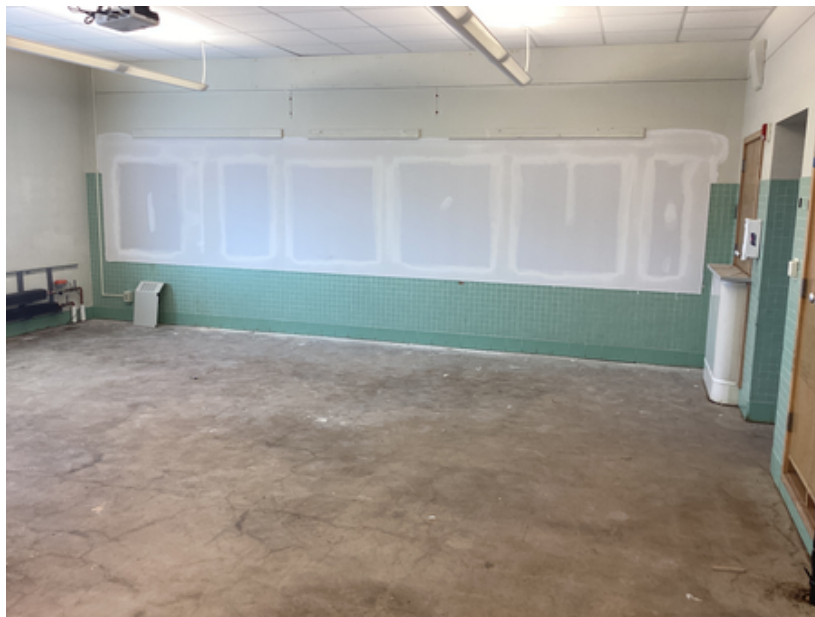
Classroom Chalkboard Removal and Wall Patching
