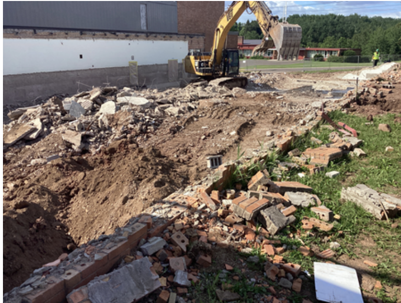
Music Suite Demolition
