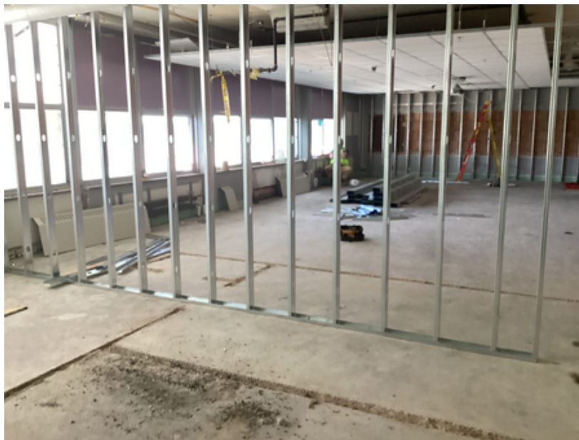
Science Rooms Wall Framing
