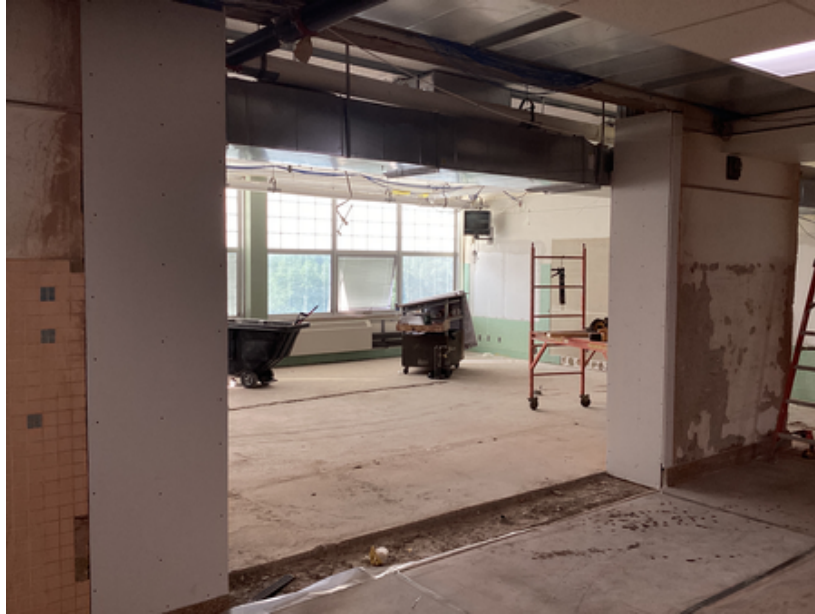
New Flex Room Openings and Progress
