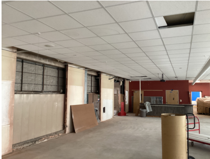
Media Center Openings and Light Removal
