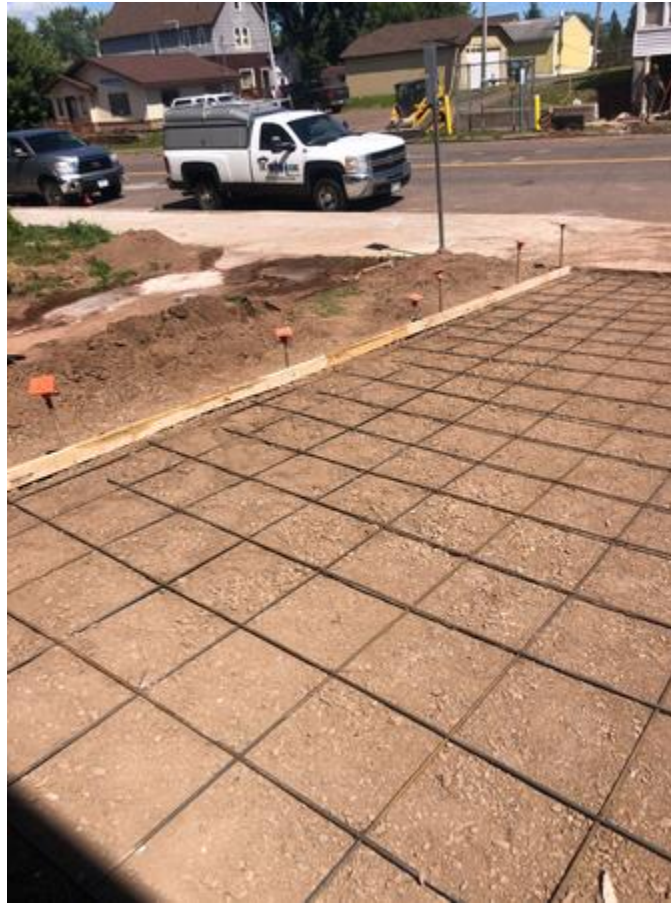
Sidewalk prep ongoing
