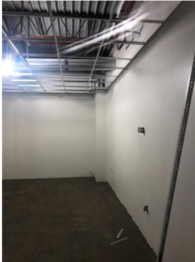
Painting, floor prep, and ceiling install ongoing throughout
