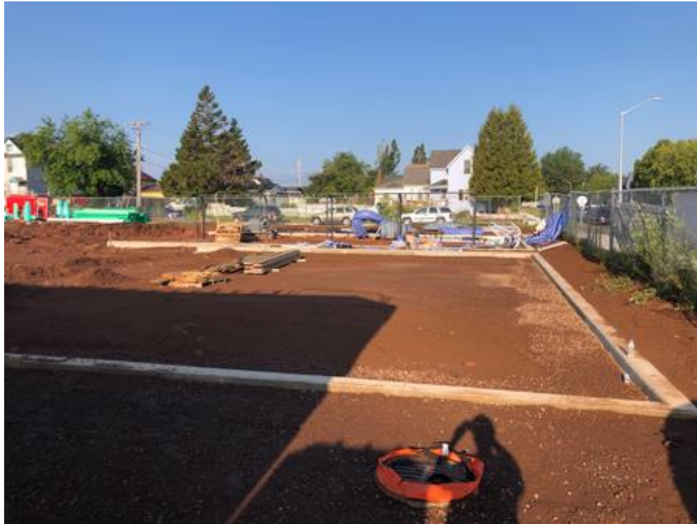
Playground equipment install ongoing
