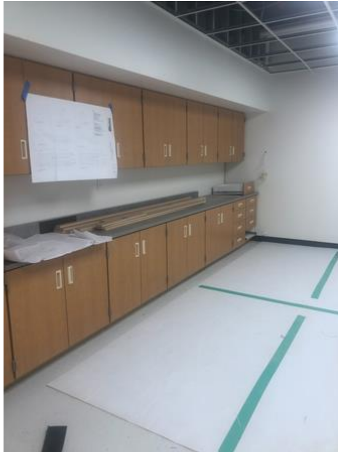
Casework install ongoing
