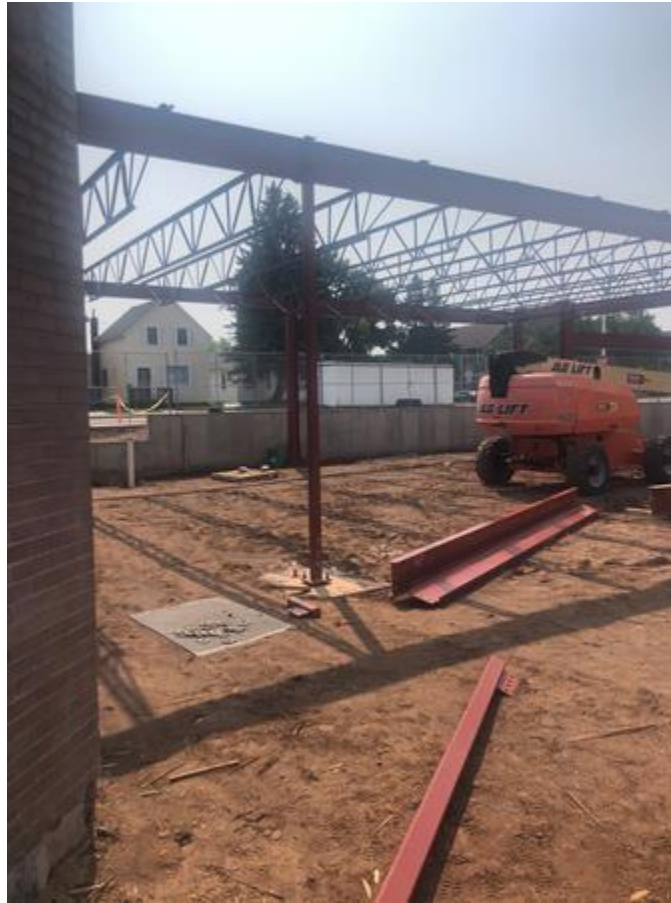
Steel erection ongoing at Cafetorium Addition
