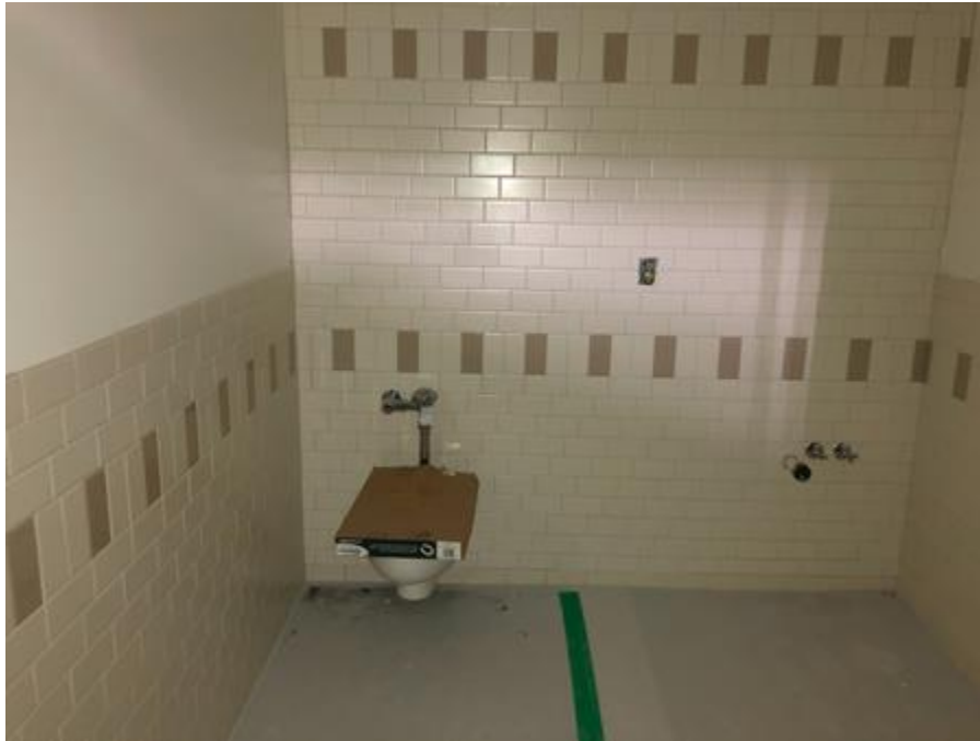
Tile and plumbing fixture install ongoing
