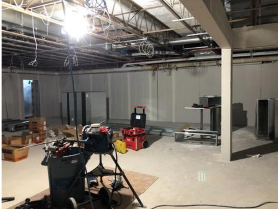
Sheetrock and taping finishing in Media Center.
