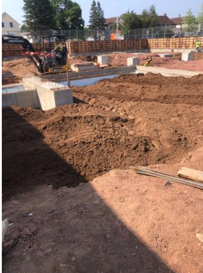
Backfilling foundation walls at Cafetorium Addition
