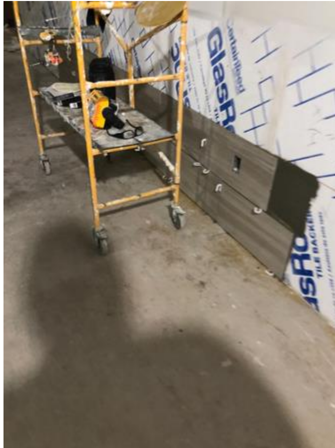
Wall Tile ongoing
