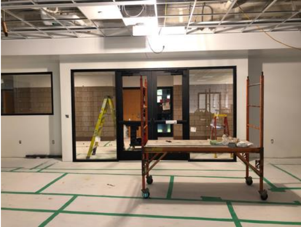
Aluminum frame installation finishing up
