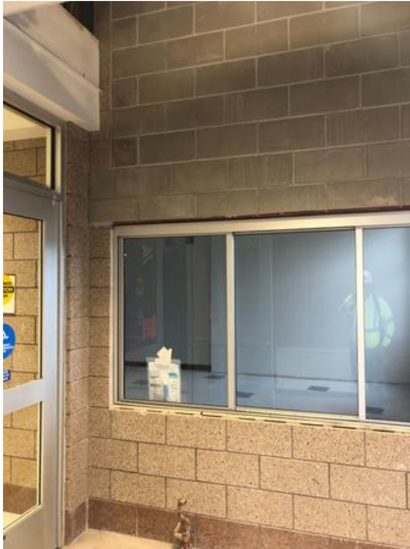
Transaction window installed
