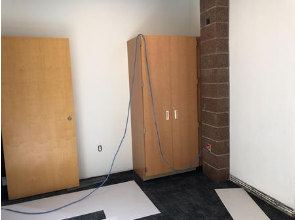
Casework, flooring and painting completed
