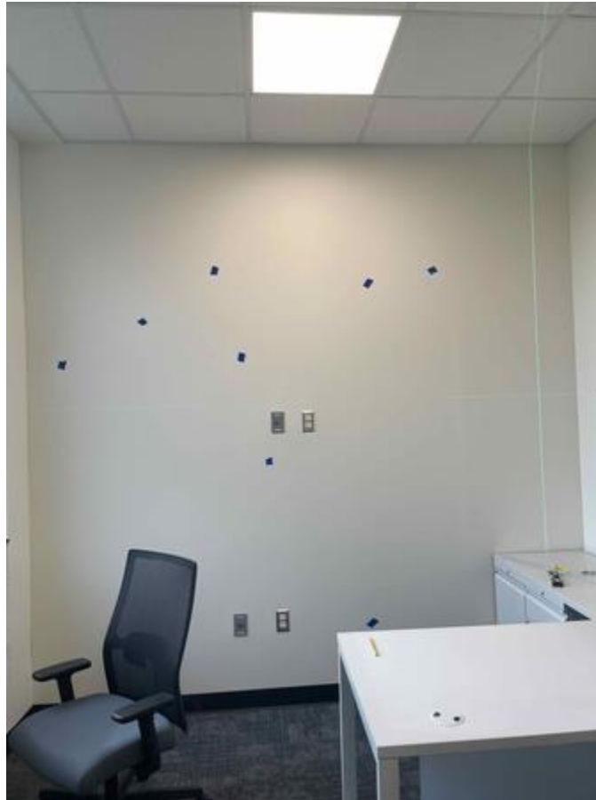
Finishes completed. Blue tape indicates punchlist items
