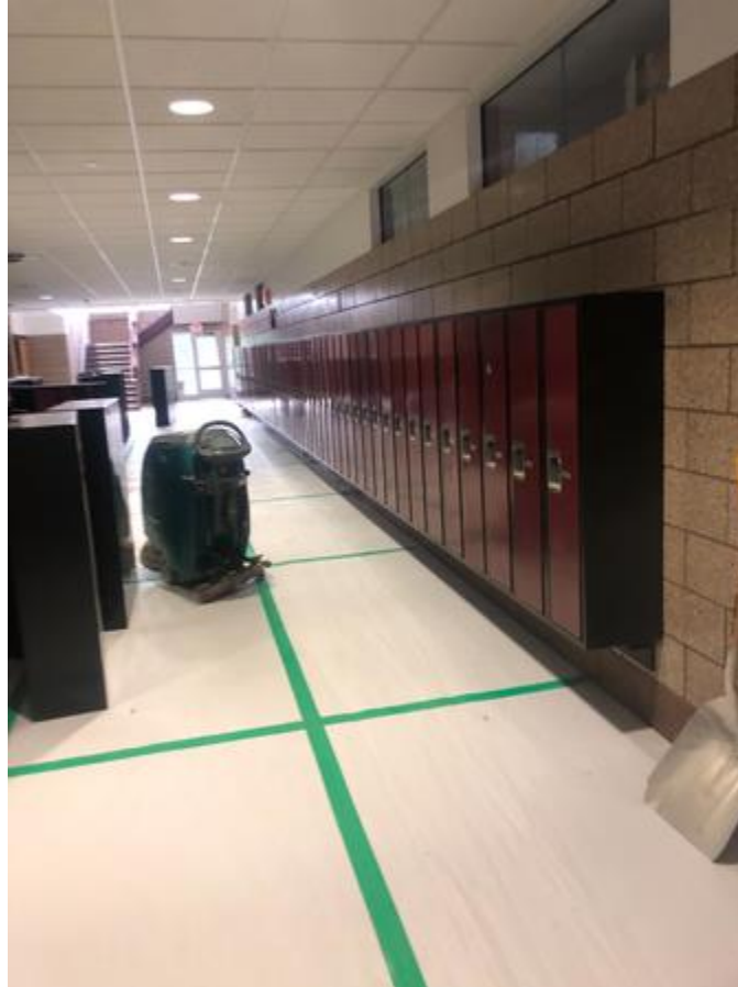
Locker install ongoing
