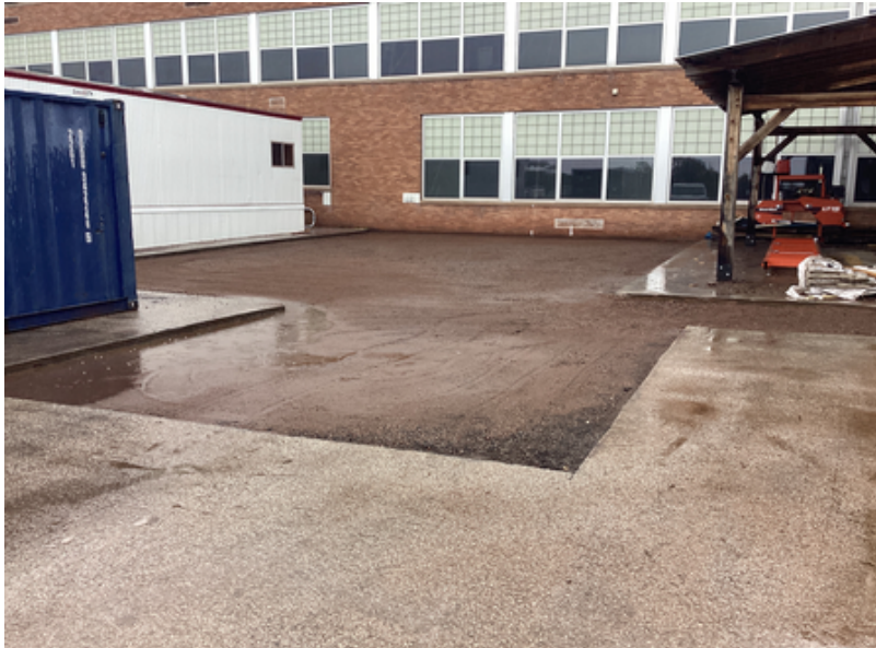
Base work for new asphalt outside of cafeteria
