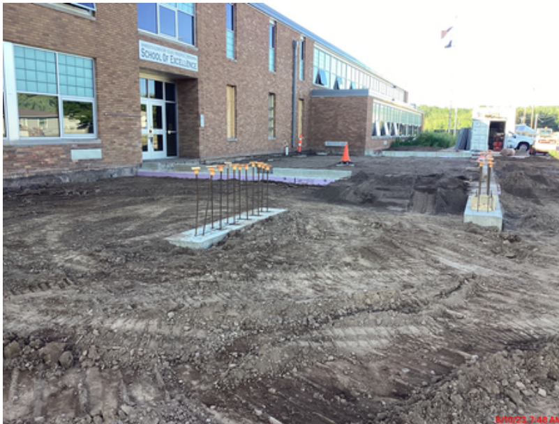
Backfilled soil for main entrance addition
