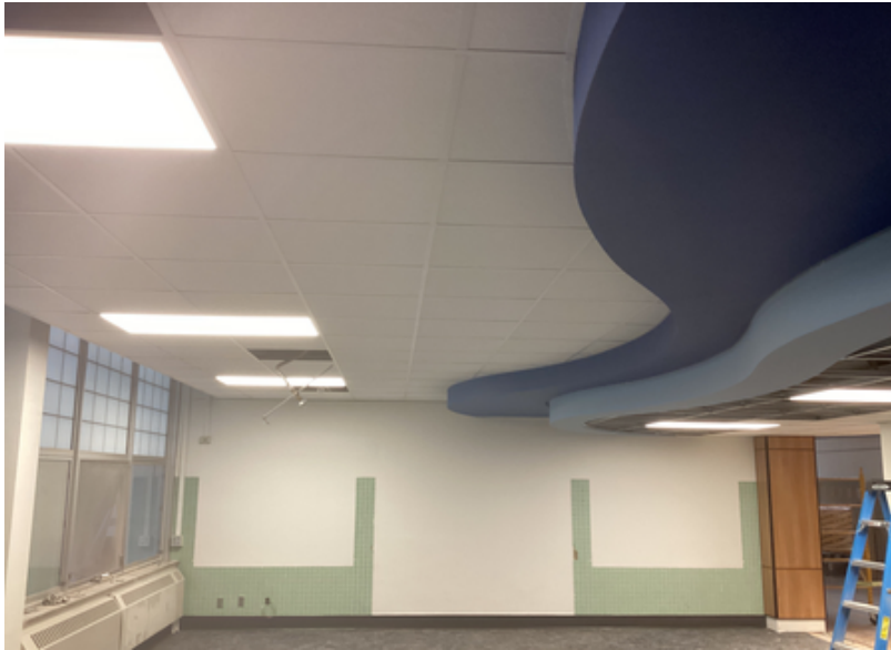
Flex Space-Carpet, Ceiling, and Light Fixtures Installed
