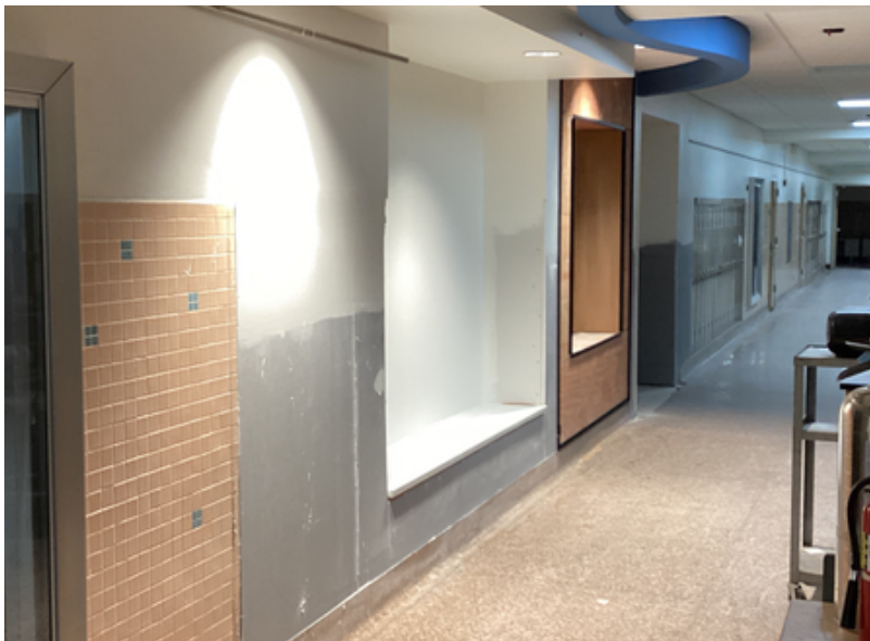
Flex Nook Corridor Space Outside Science Classrooms
