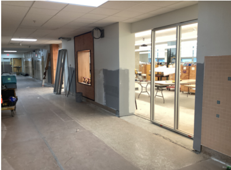
Media Center Corridor Interior Glass Installation
