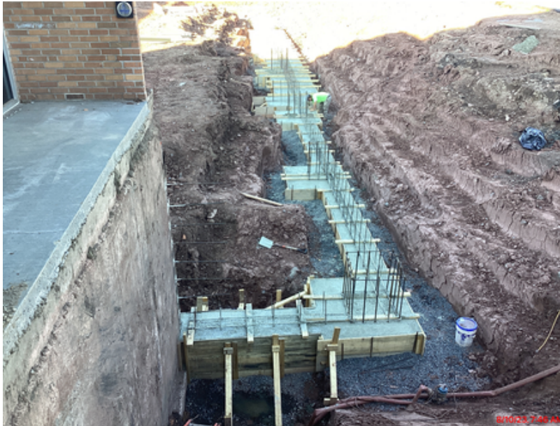
Footings and foundations at Music Suite addition
