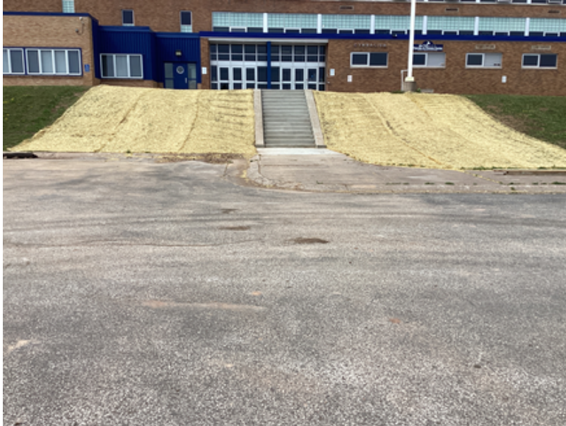
Seed blankets for grass at new concrete stairs
