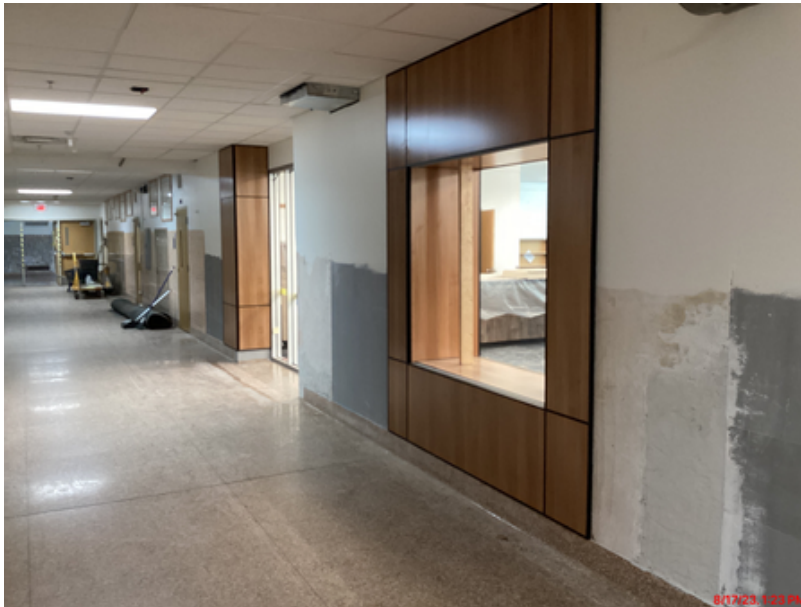
Media Center Corridor Interior Glass Installation
