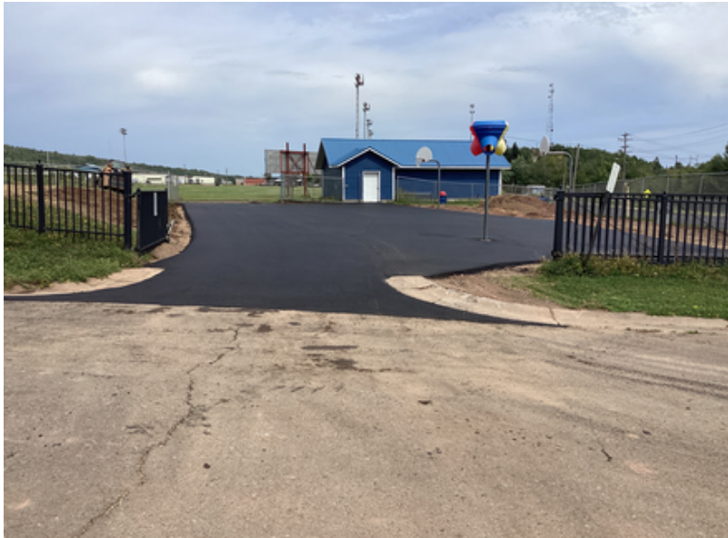
New asphalt pavement at basketball playground
