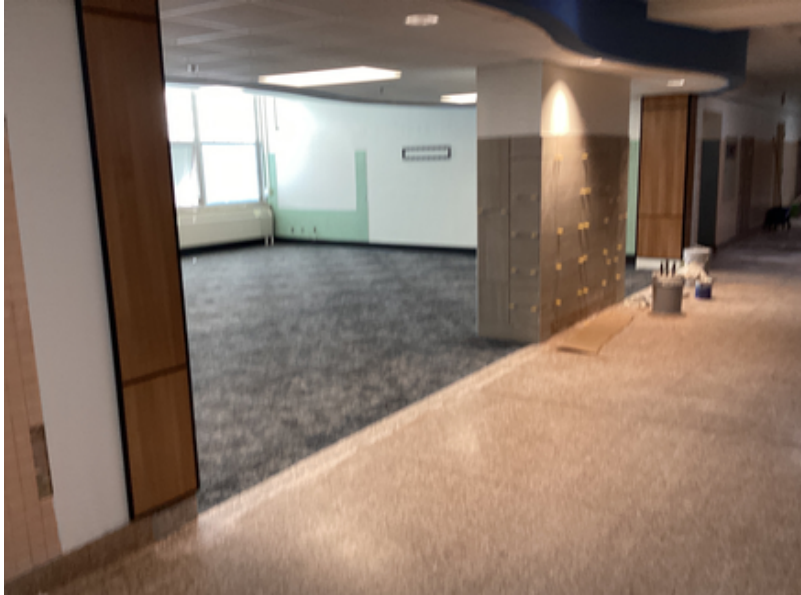
Flex Space Entrance – Wall Tile
