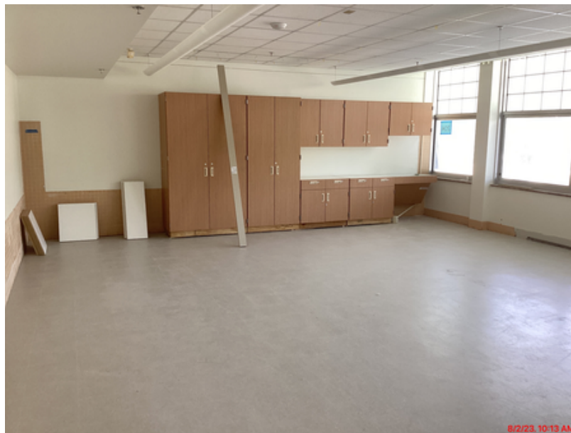
Classroom casework installation
