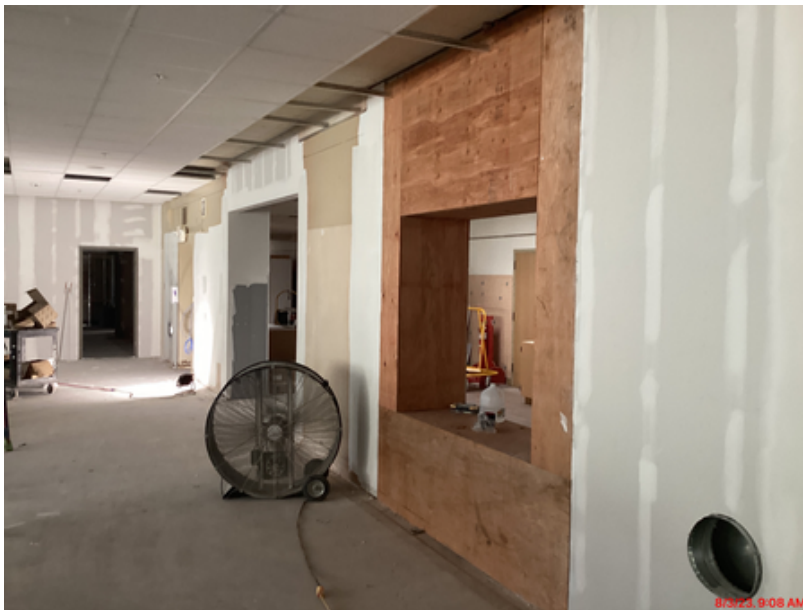
Media Center drywall and display case framing
