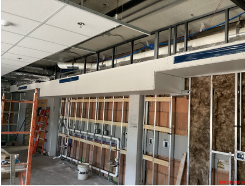
Science Classrooms plumbing and electrical rough ins.
