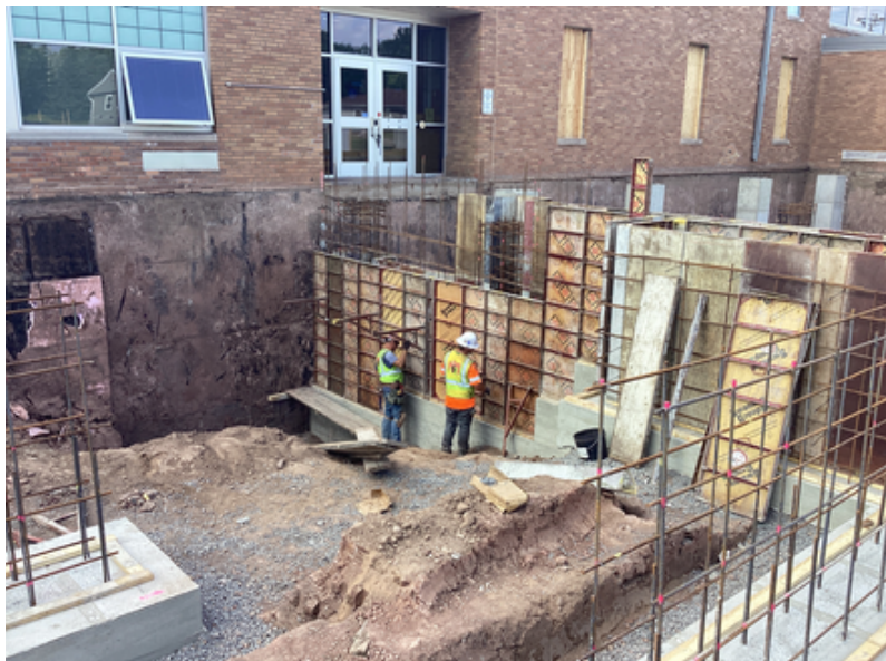
Forming walls for main entrance addition
