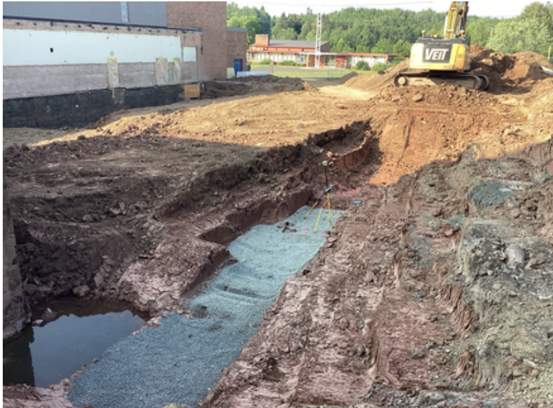
Excavation for footings and foundations at Music Suite addition
