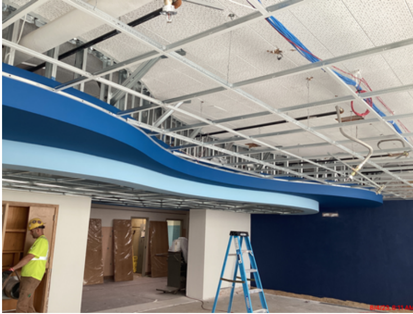
Ceiling grid installation in new flex space
