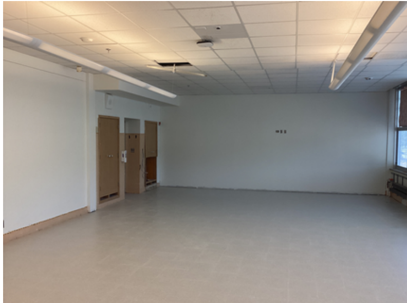
Flooring and painting in classrooms
