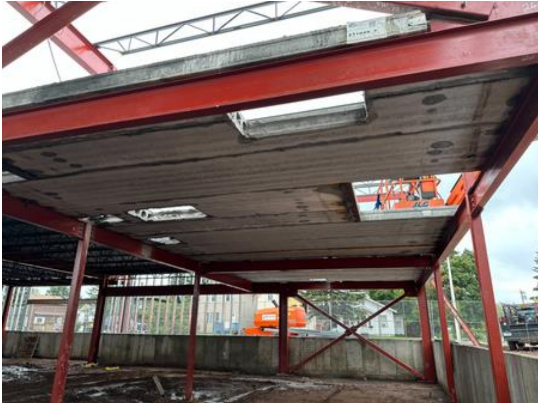
Precast plank completed
