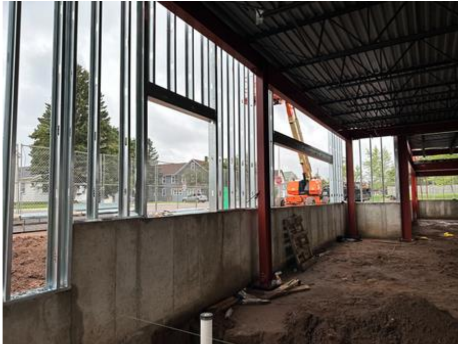
Exterior steel stud framing ongoing
