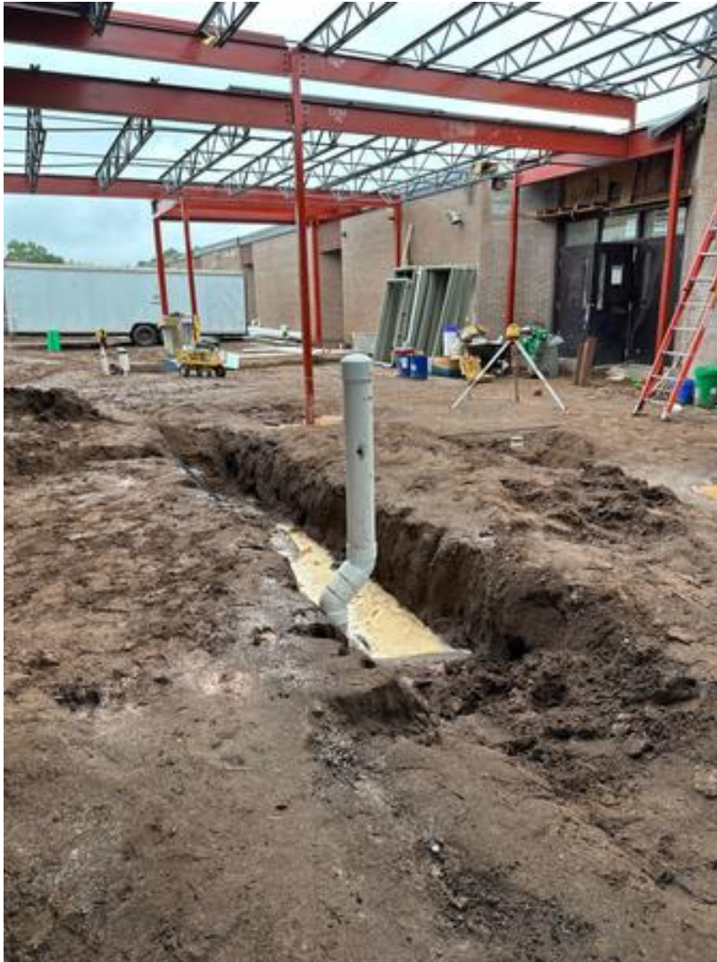
Underground plumbing ongoing
