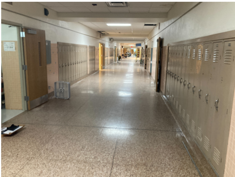
Corridors cleared and cleaned
