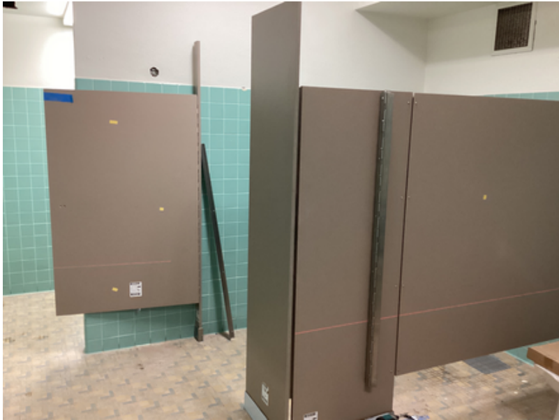
Toilet partition installation
