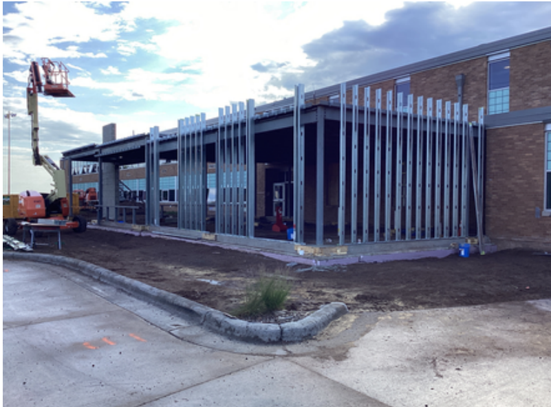
Exterior wall framing at new main entrance
