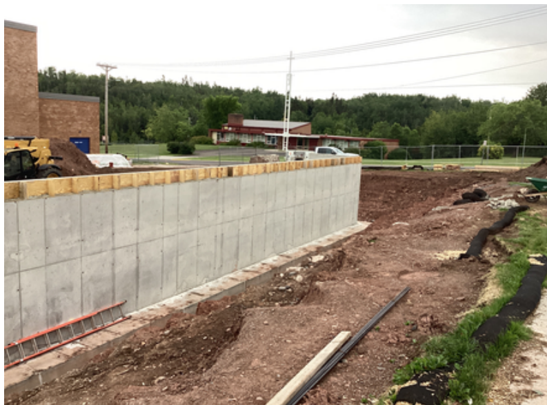
Music Addition north wall foundation poured
