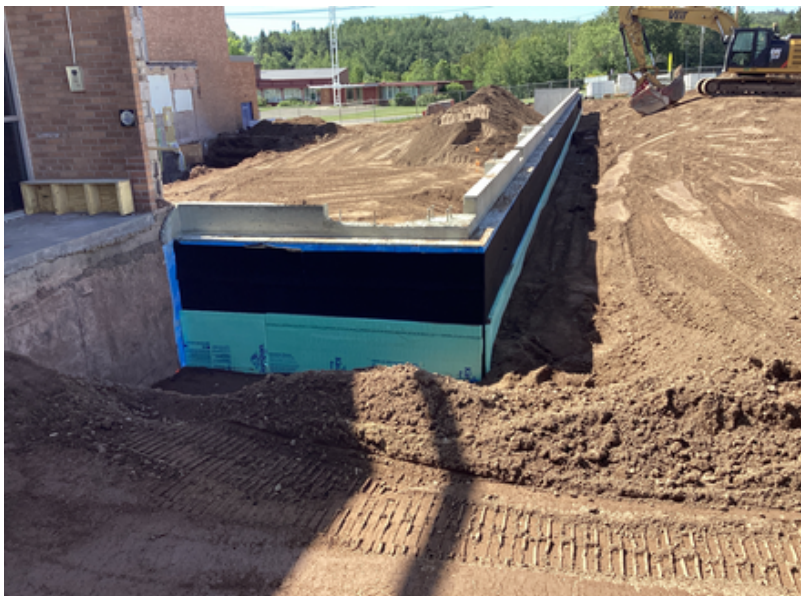
Music Addition Water Proofing and Insulation
