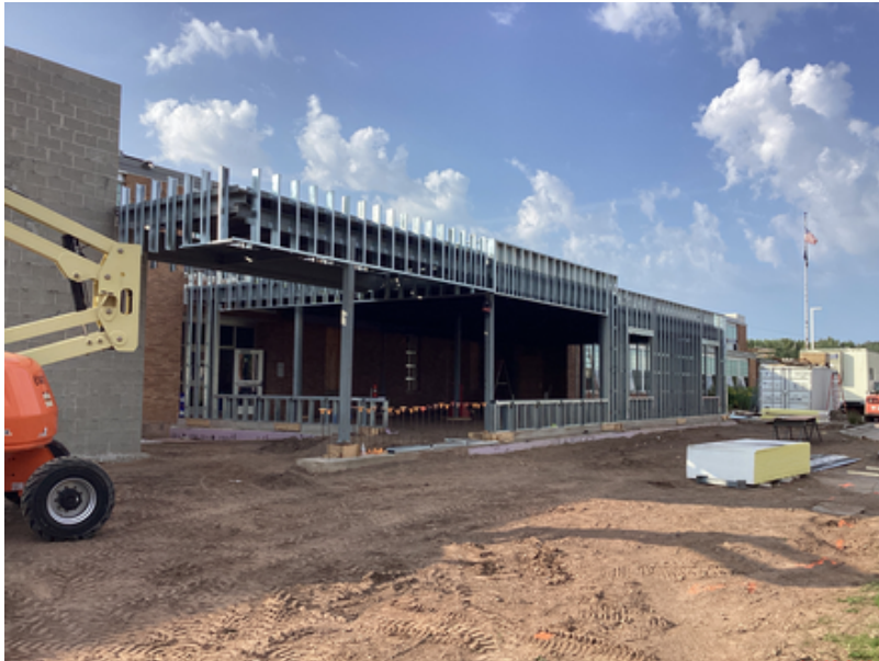
Exterior wall framing at new main entrance
