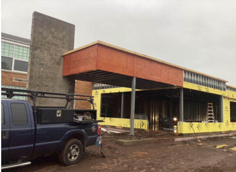
Canopy framing at main entrance
