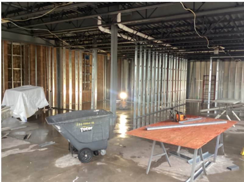
Concrete floor poured and wall framing at main entrance addition/administration offices
