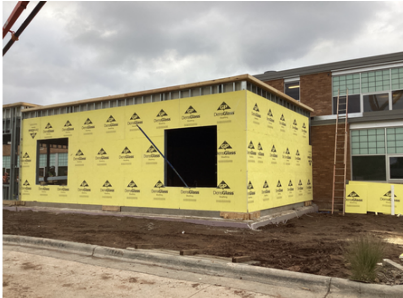
Exterior wall framing at new main entrance
