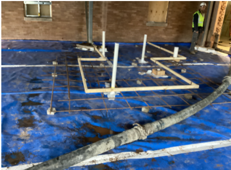
Plumbing and rebar at main entrance
