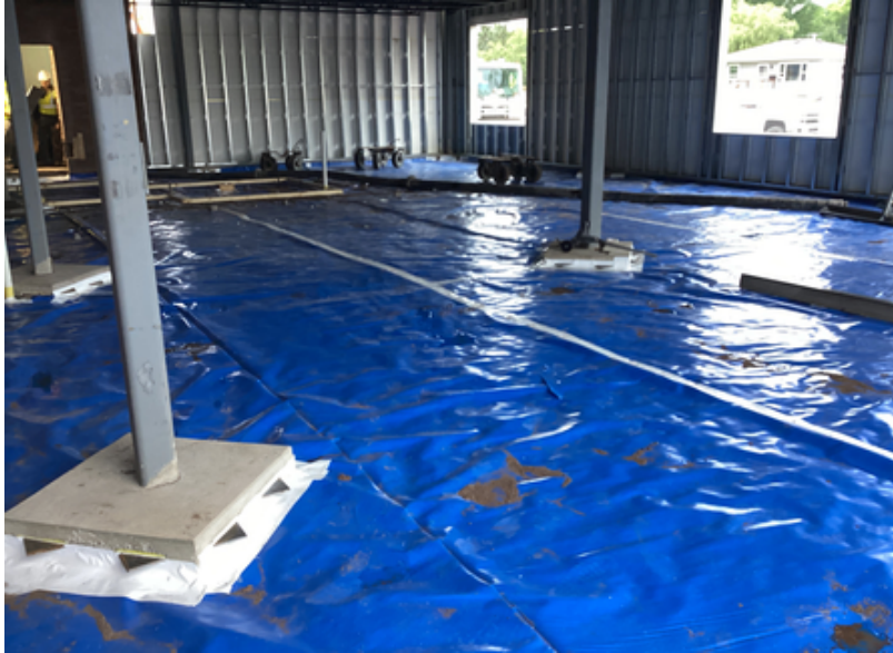
Vapor Barrier and concrete floor preparation at main entrance
