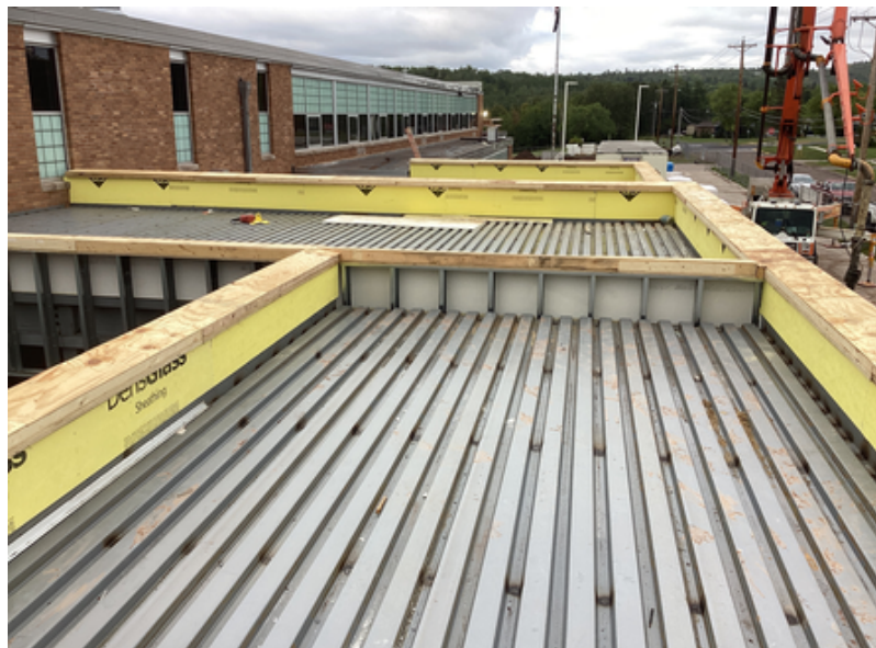
Roof blocking and parapets at main entrance
