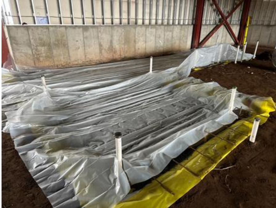
Freezer/cooler pad poured
