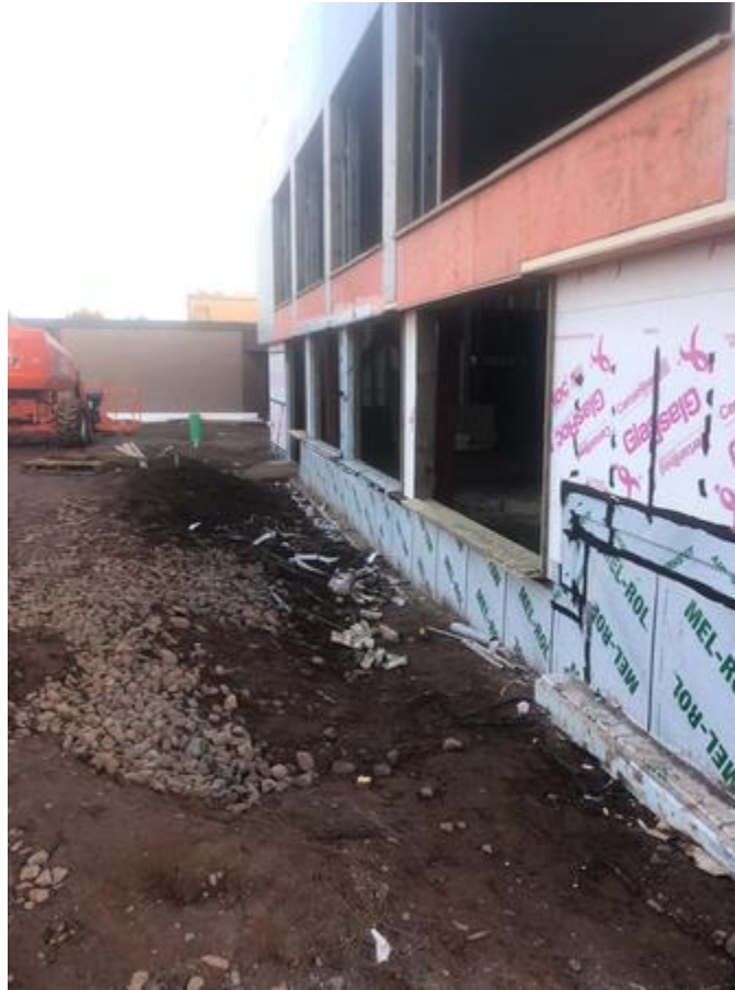
Exterior sheathing, weather barrier, and window blocking ongoing
