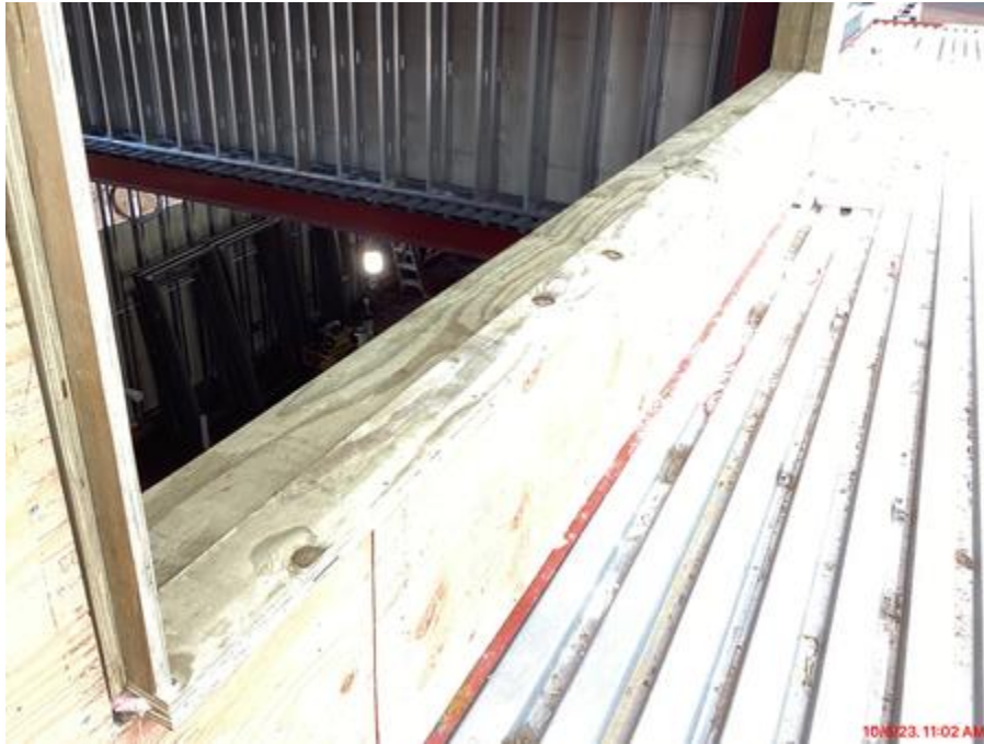
Window blocking ongoing
