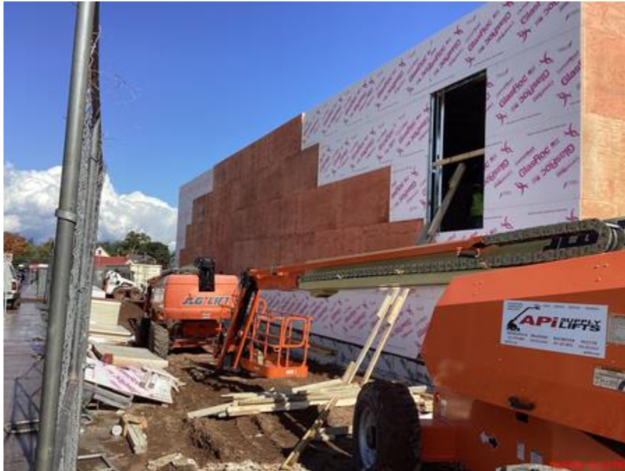
Exterior sheathing and plywood installation ongoing
