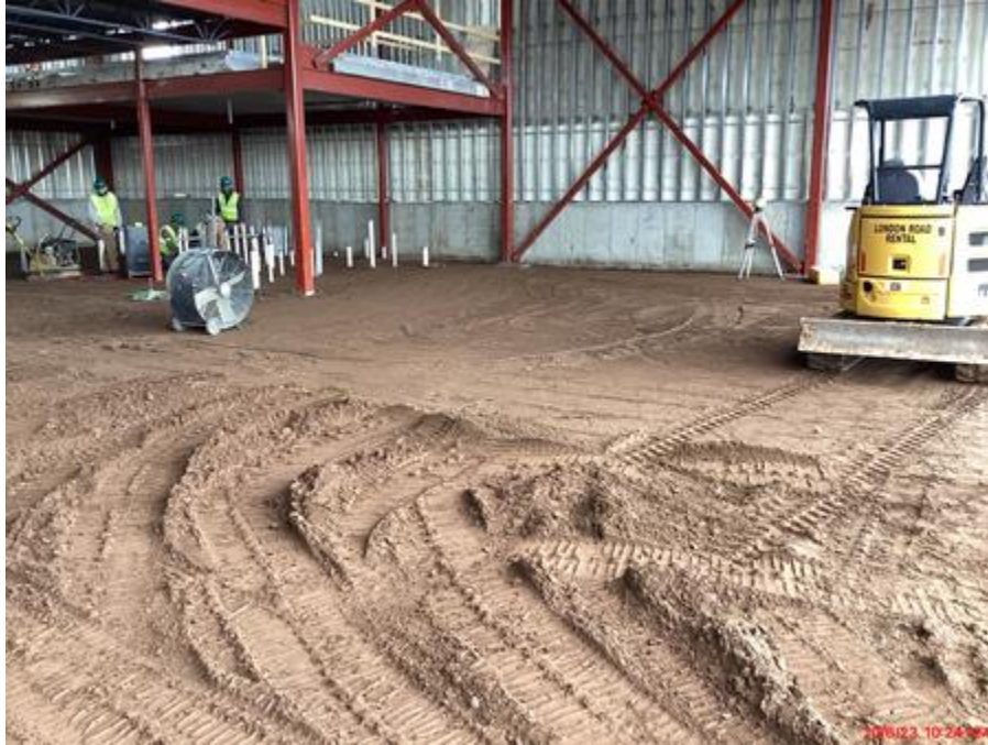
Underground plumbing and electrical complete. Sand cushion being installed
