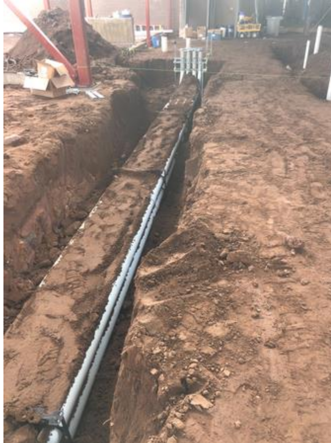
Underground electrical ongoing
