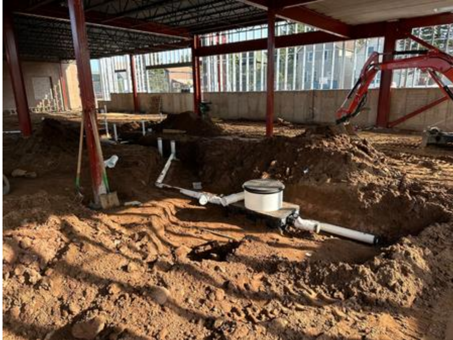
Underground plumbing ongoing for kitchen area
