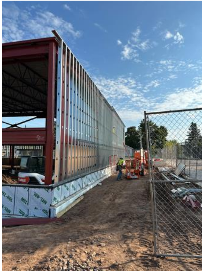
Exterior steel stud framing ongoing
