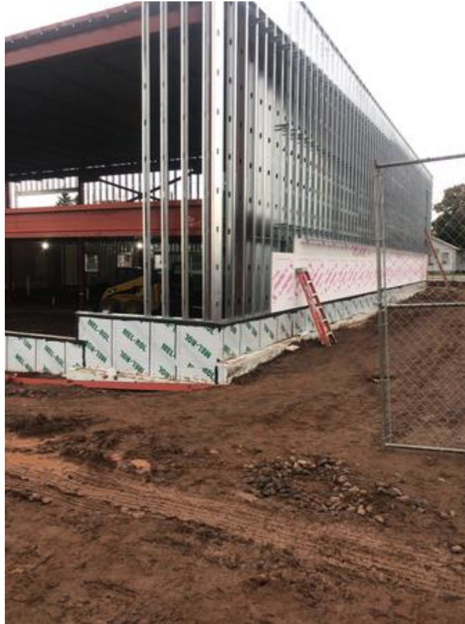
Exterior steel stud framing and sheathing ongoing
