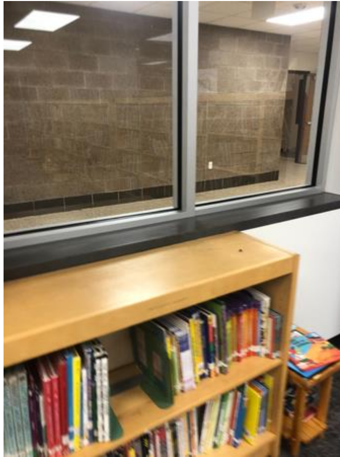
Interior window sills ongoing
