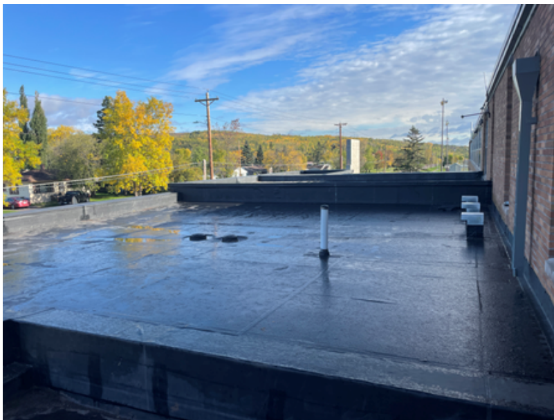
Roof work at main entrance addition.
