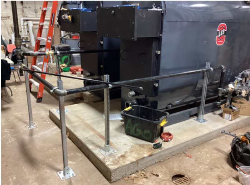
Boilers' piping installation
