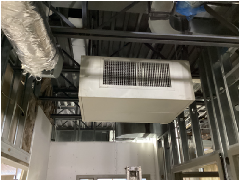
Wall framing and mechanical equipment installation at main entrance addition
