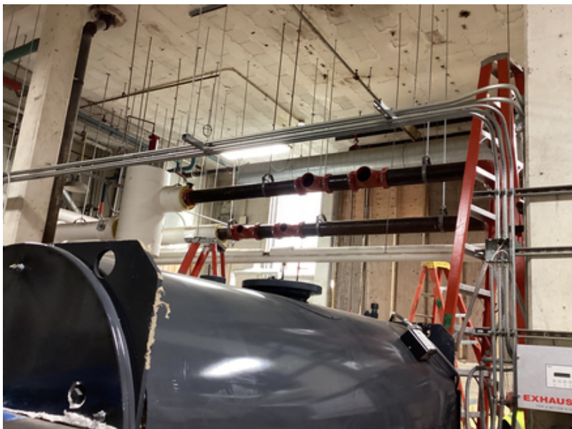
Boilers' piping installation
