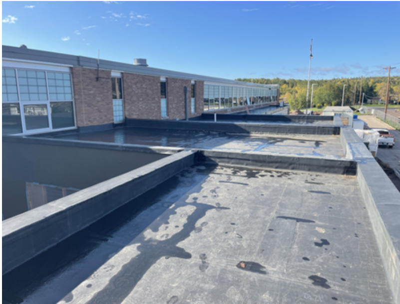
Roof work at main entrance addition.
