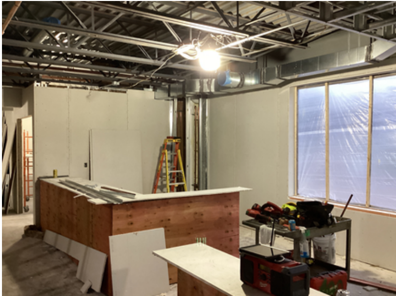
Wall framing and mechanical/electrical rough ins at main entrance addition
