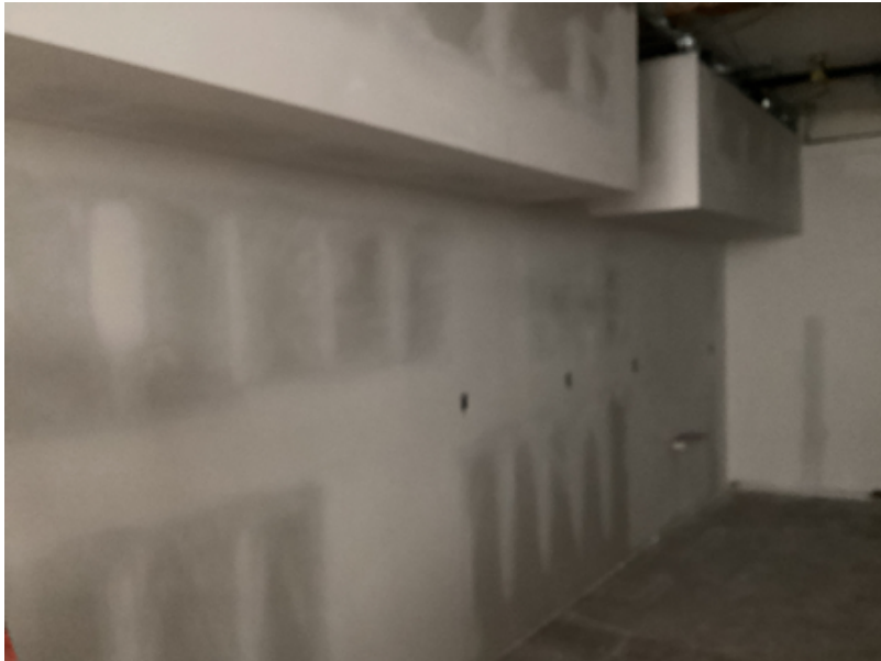
Taping and mudding drywall at main entrance addition
