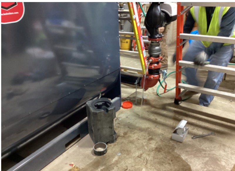
Boilers' piping installation
