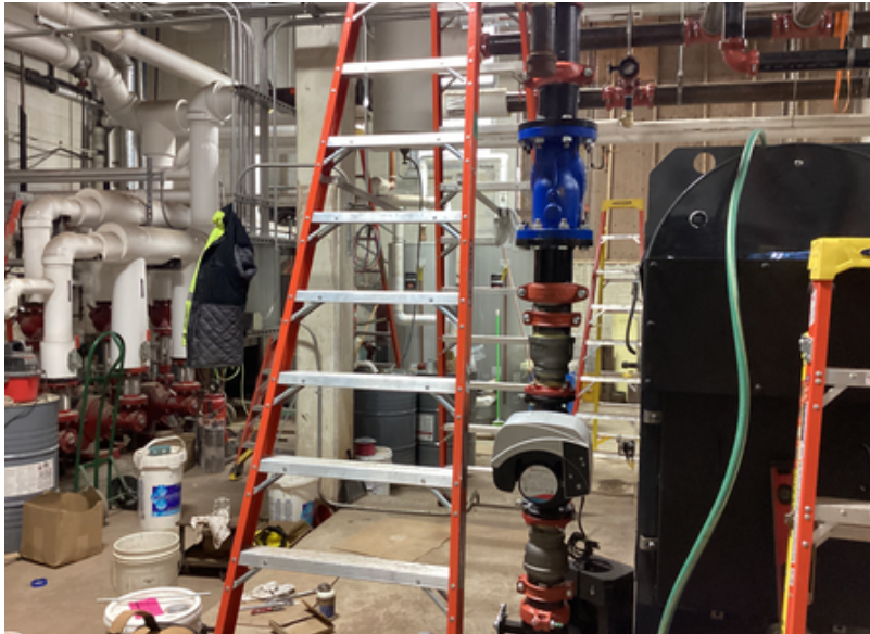
Boilers' piping installation
