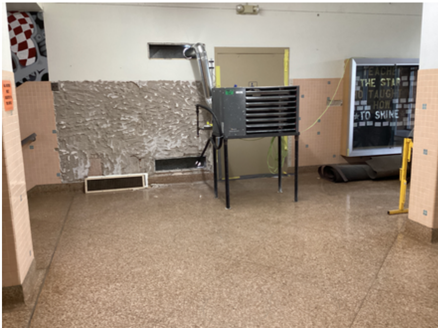
Temporary heating units installation
