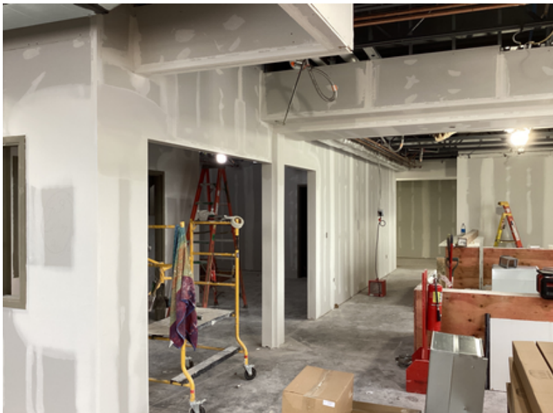
Main Entrance drywall taping and mudding
