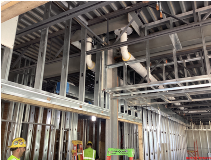
Wall framing and mechanical/electrical rough ins at main entrance addition
