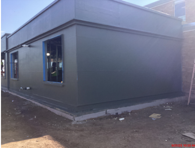
Weather proofing on main entrance addition
