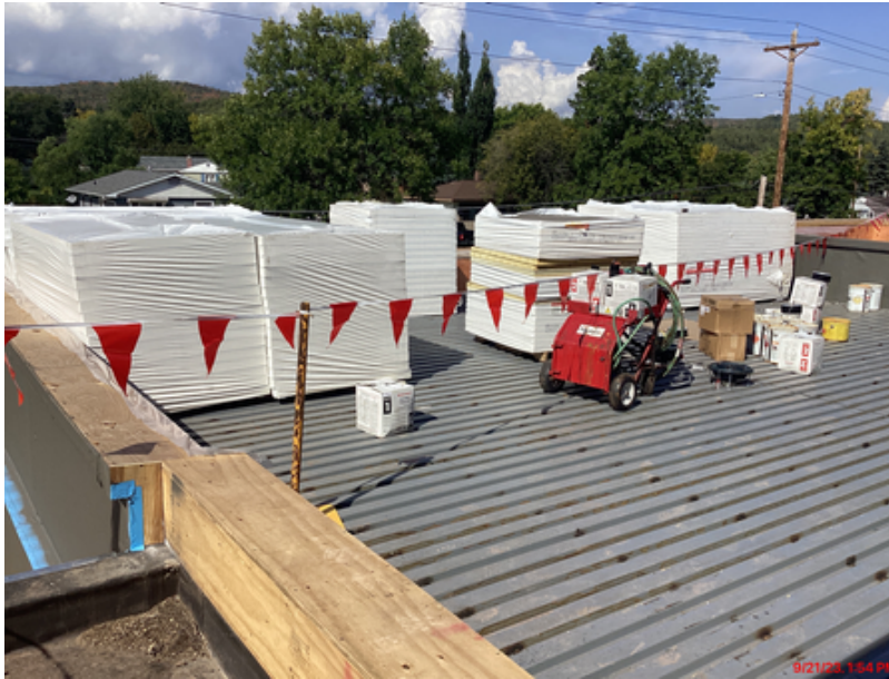
Roof work and staging at main entrance addition.
