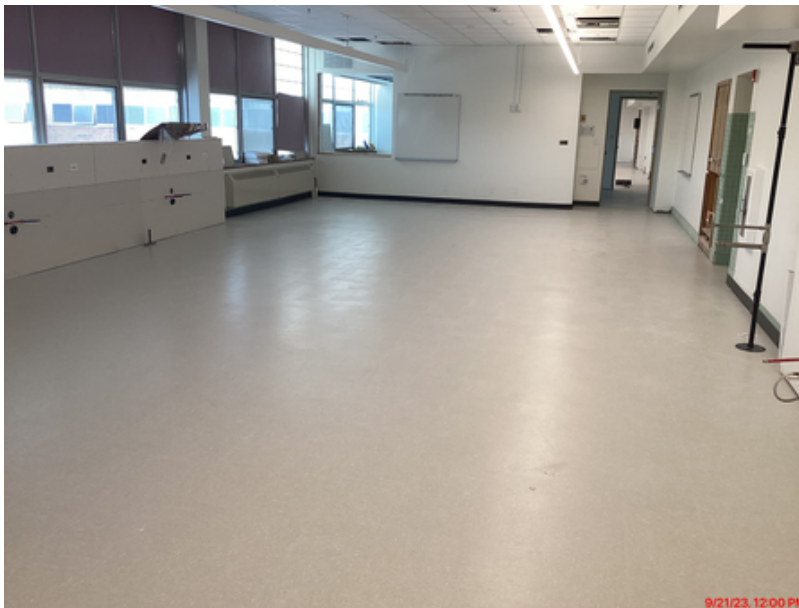
Flooring installation in Science Rooms
