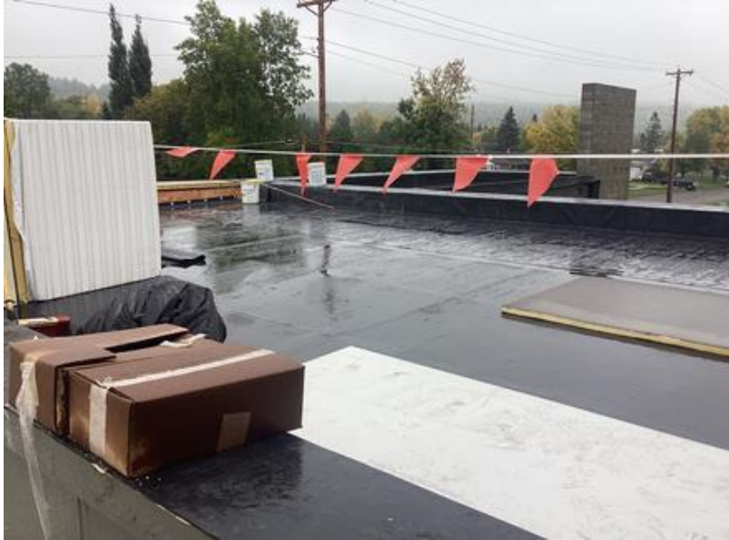
Roof work and staging at main entrance addition.
