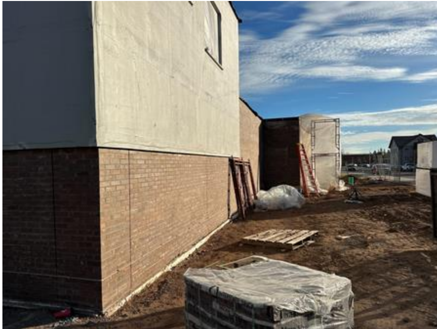
Brick installation ongoing
