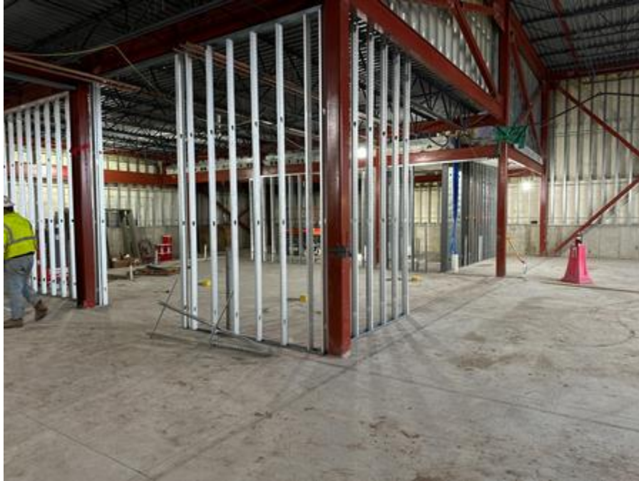
Interior Steel Stud Framing ongoing
