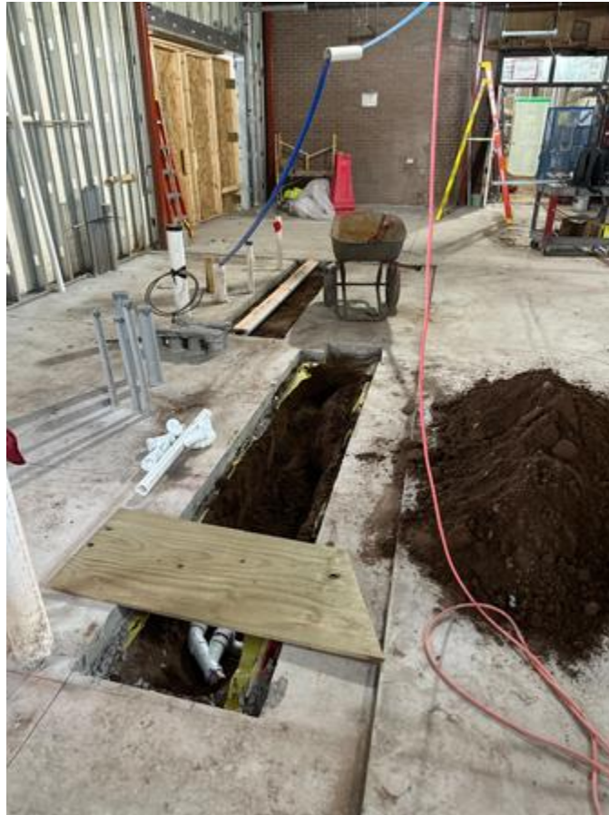
Floor drain rough-ins ongoing for restroom area
