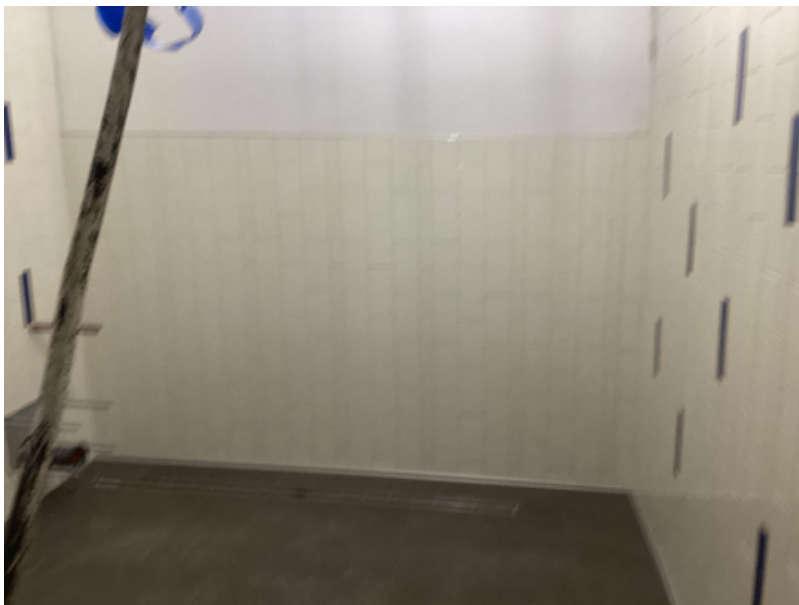
Tile work at new Main Entrance
