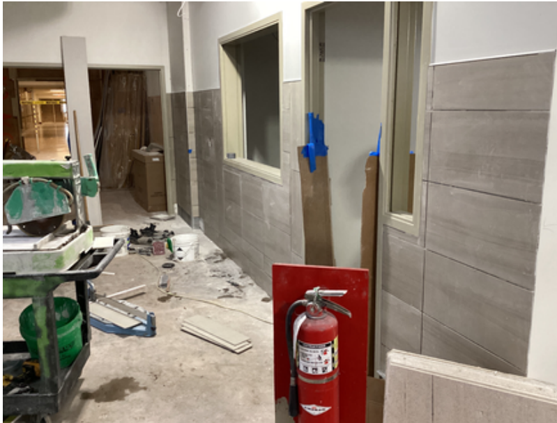
Tile work at new Main Entrance
