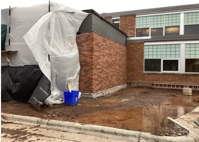
Brick installation at New Main Entrance
