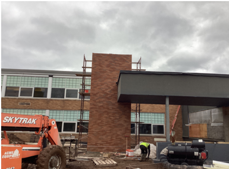
Brick installation at New Main Entrance
