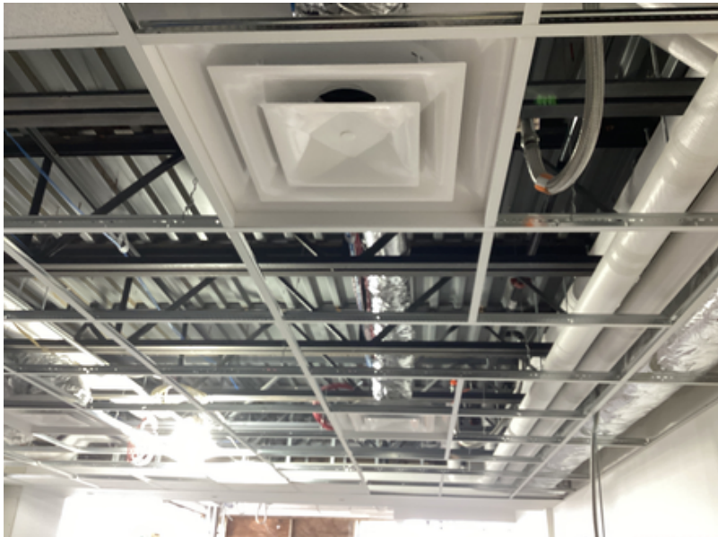
Ceiling work at New Main Entrance
