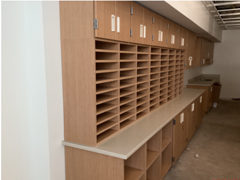
Casework Installation at New Main Entrance
