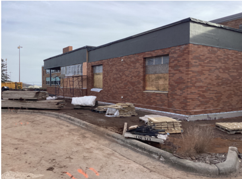
Brick installation at New Main Entrance
