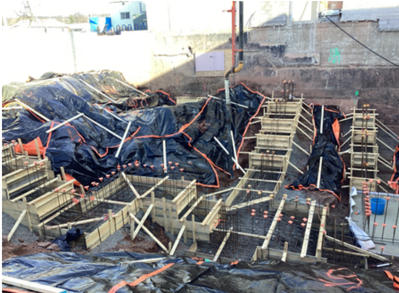
Forms for footings at Area B Music Suite
