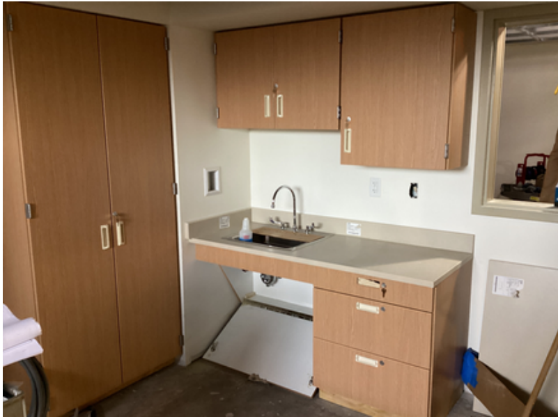
Plumbing/Casework Installation at New Main Entrance
