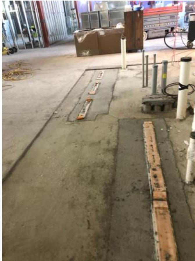
Floor drains installed and concrete poured back
