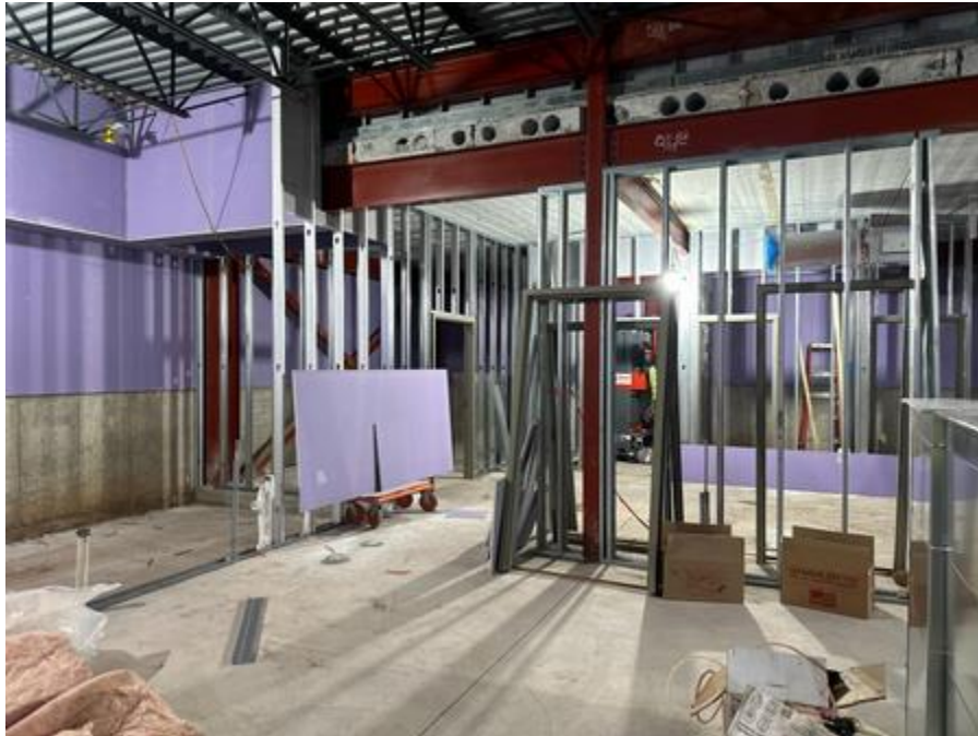
Interior framing, spray foam and sheetrock ongoing
