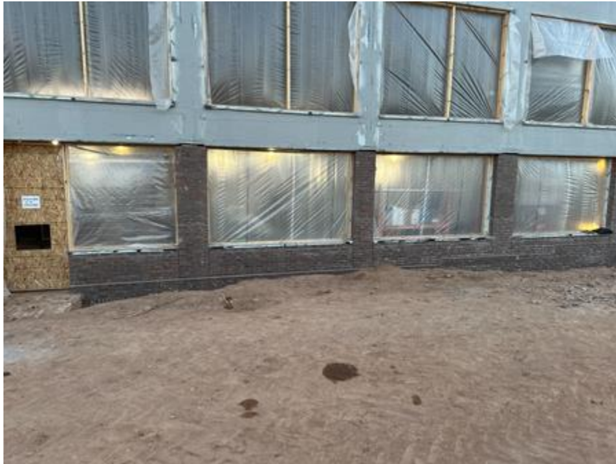
Exterior brick finishing up, exterior metal panels to follow
