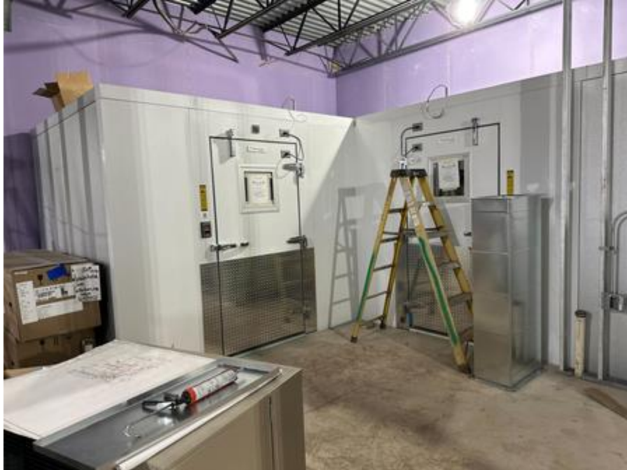
Freezer and Cooler installed
