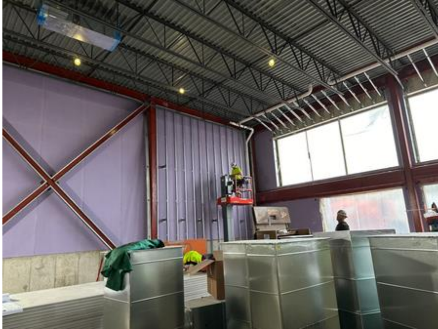
Sheetrock and framing ongoing
