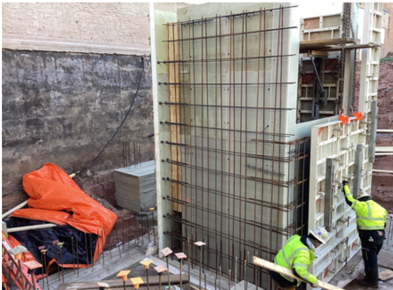
Music Suite Elevator Wall Forms
