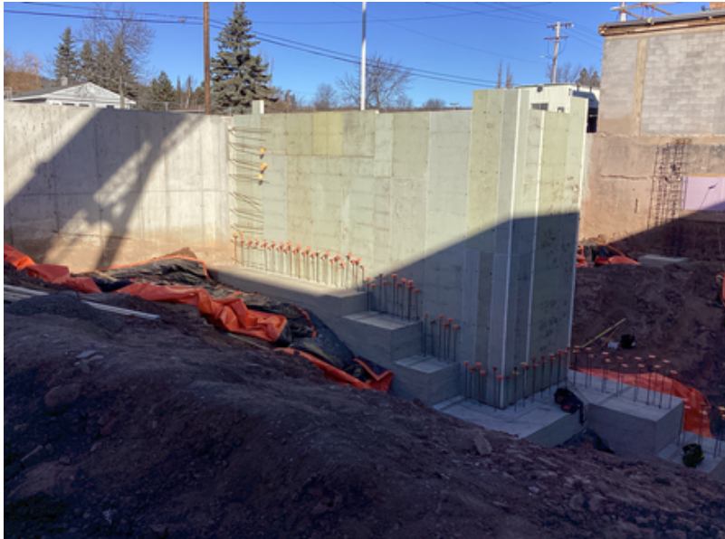
Footings at Area B Music Suite
