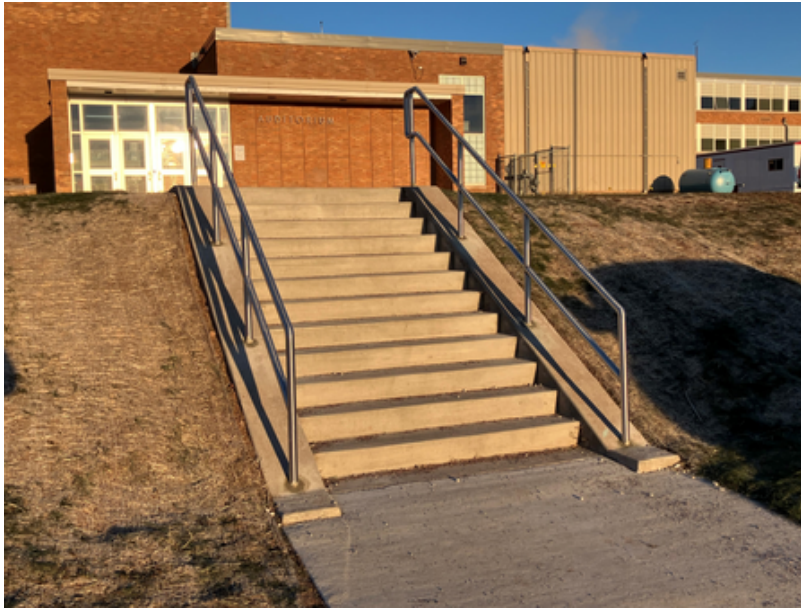
Exterior Handrails Installed
