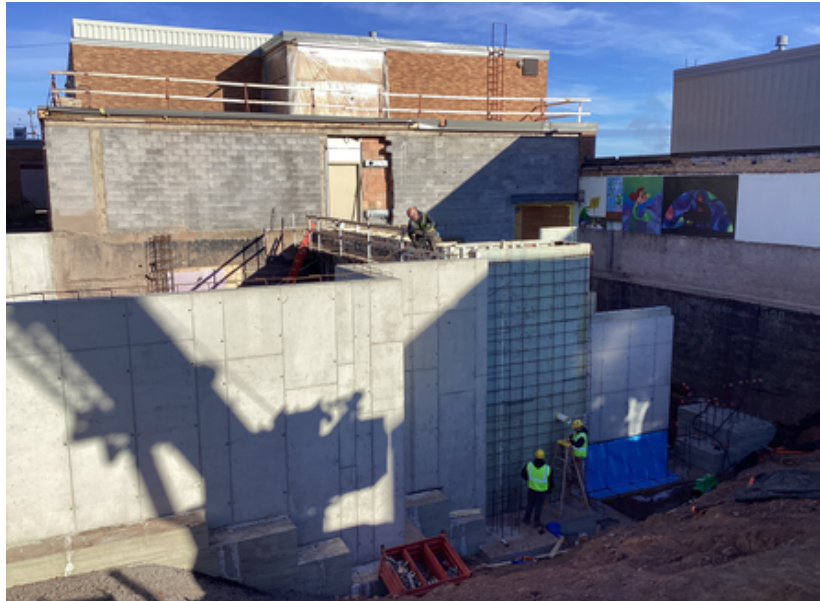
Foundation Walls at Area B Music Suite
