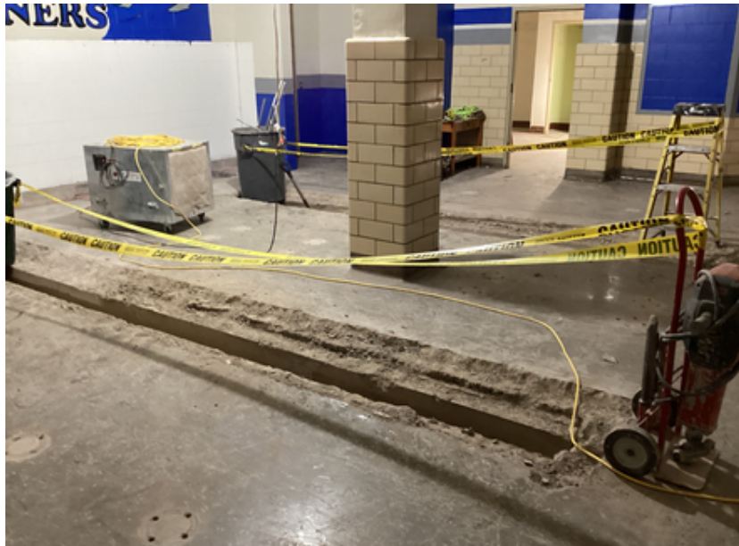
Boy Locker Room Demolition
