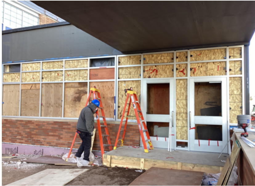
Aluminum Storefront at Main Entrance
