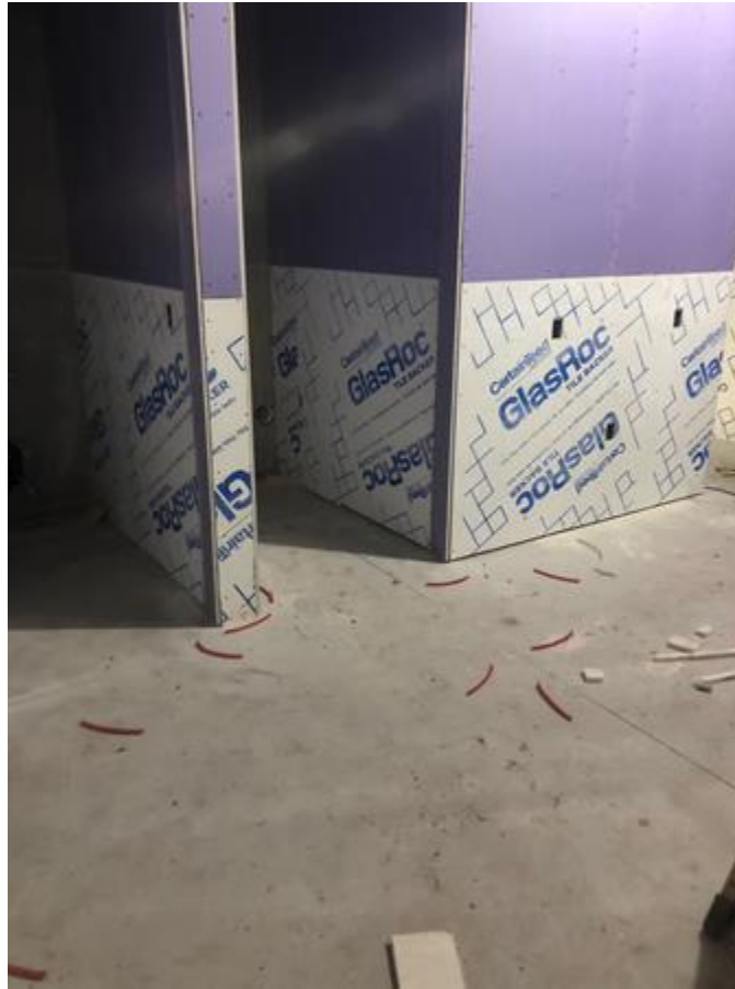
Restrooms ready for tile installation
