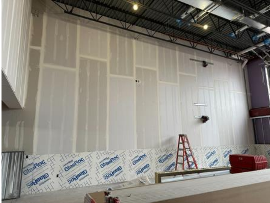
Sheetrock and taping ongoing
