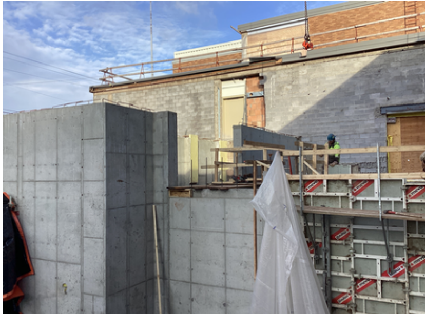
Foundation Walls and elevator shaft wall at Area B Music Suite
