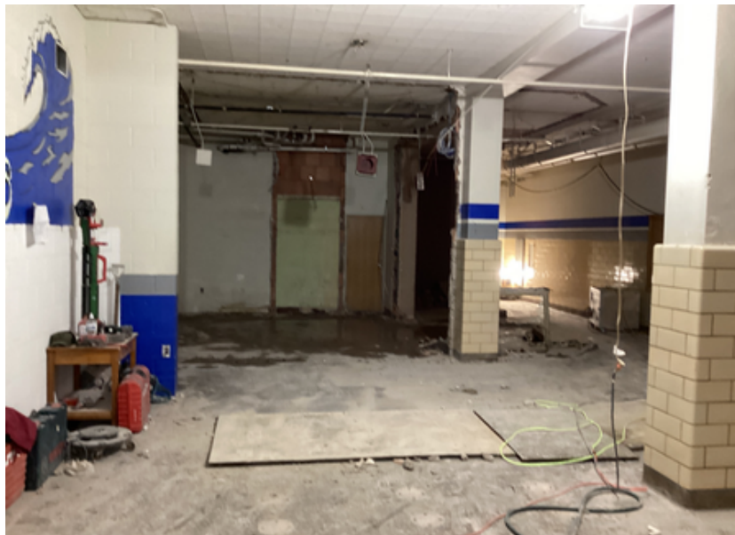
Boy Locker Room Demolition
