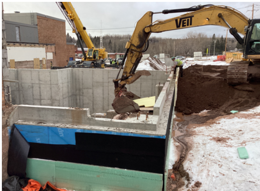
Backfilling soils at Area B Music Suite
