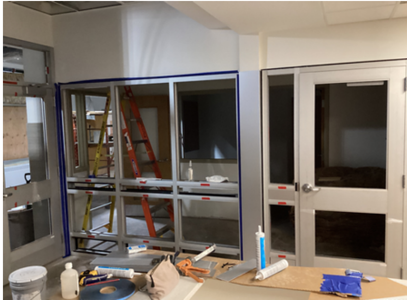
Interior Vestibule Aluminum Storefront at Main Entrance
