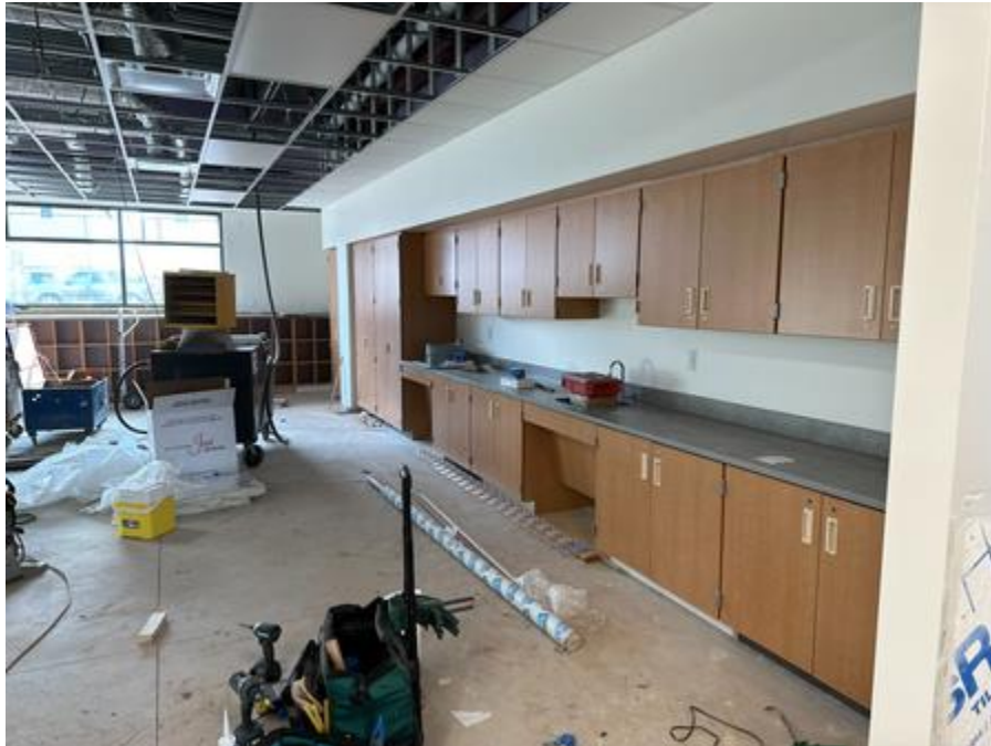
Casework installation ongoing
