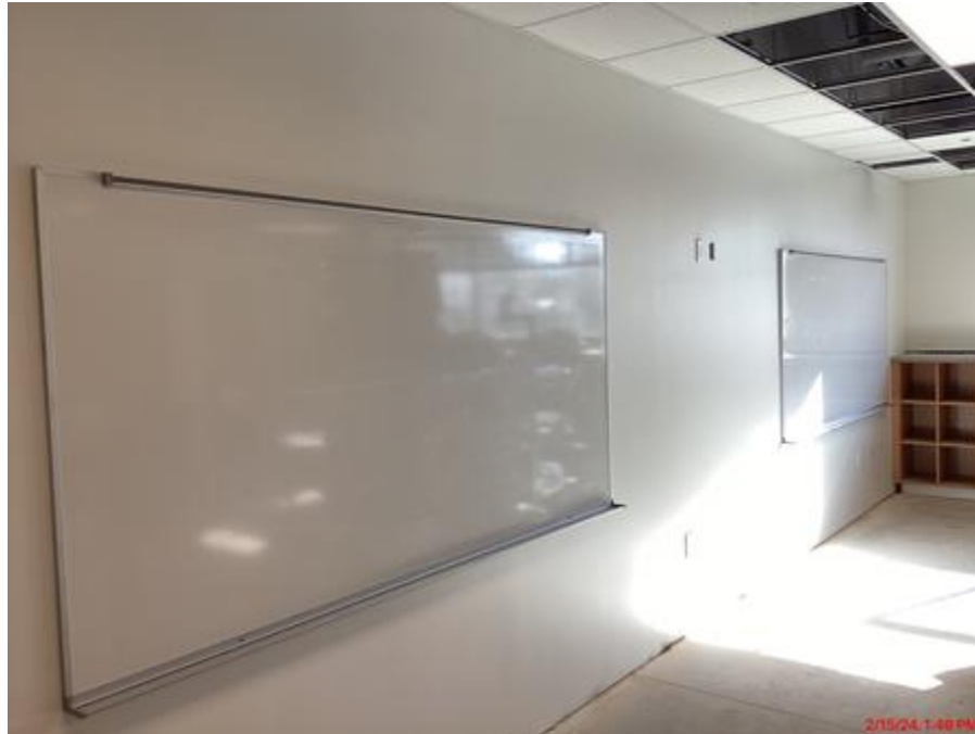
Markerboard installation ongoing
