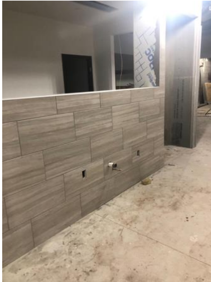
Hallway and bathroom tile finishing up
