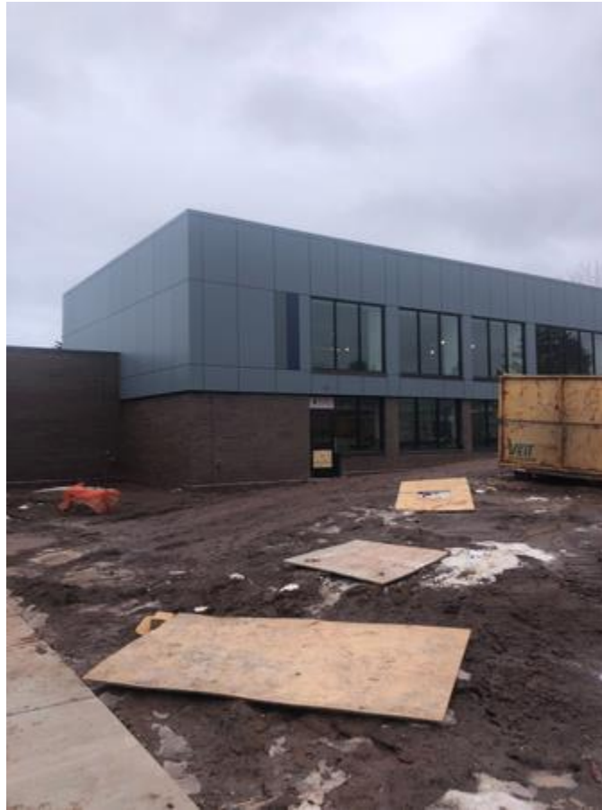
Exterior Metal Panels finishing up
