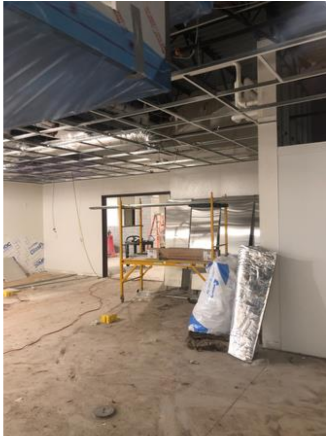
Ceiling grid installation ongoing
