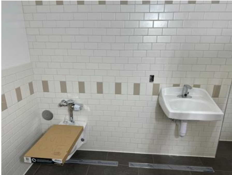
Setting plumbing fixtures
