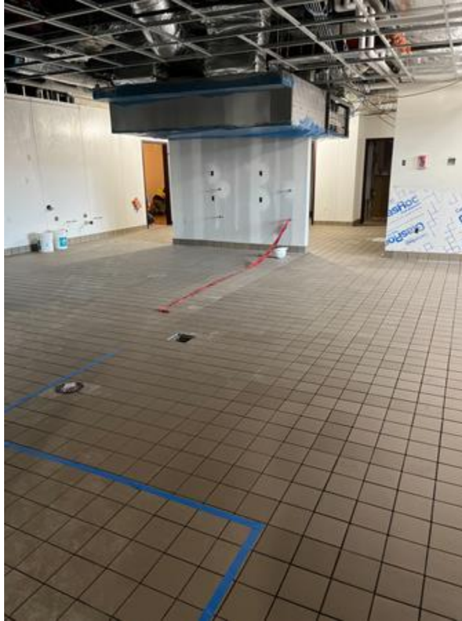
Tile in kitchen ongoing
