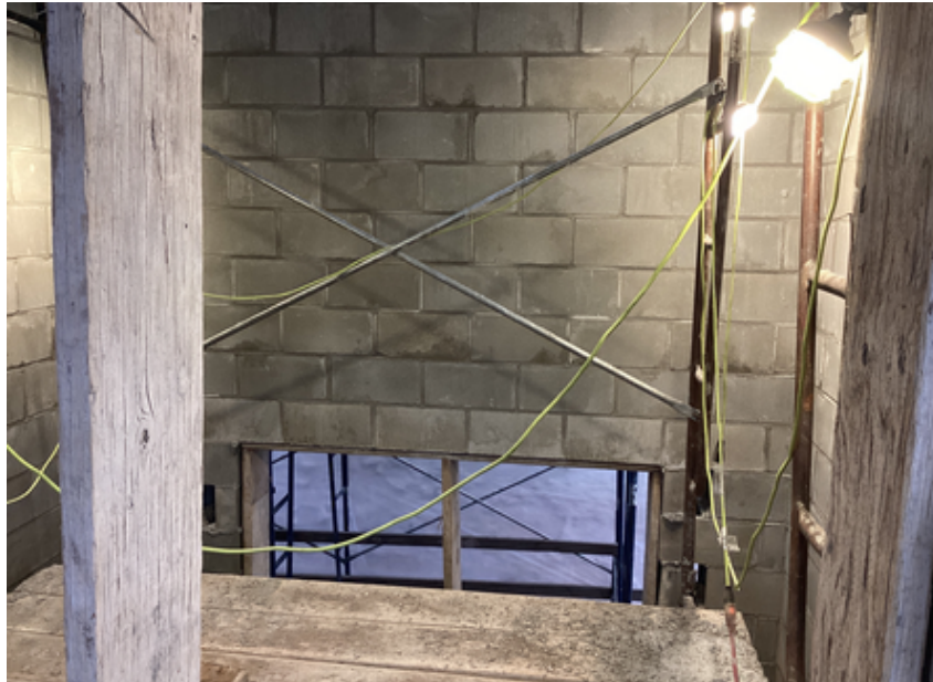
Elevator walls at Area B Music Suite
