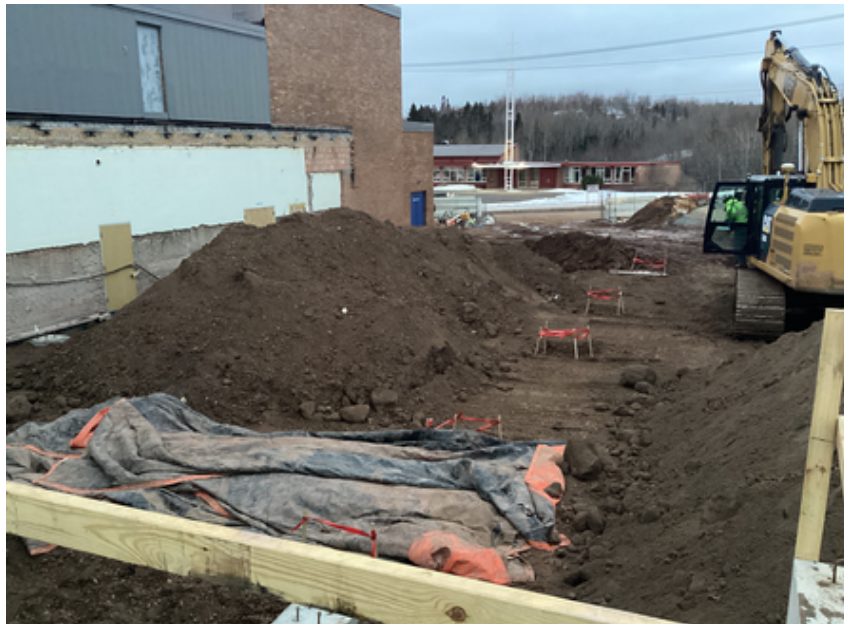
Backfilling Area B Music Suite
