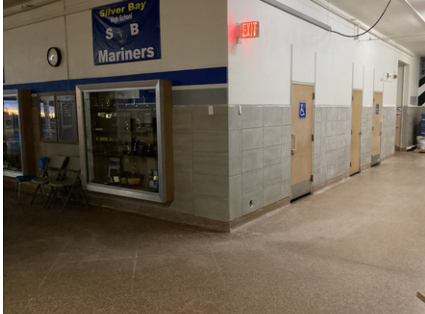
Corridor tile work
