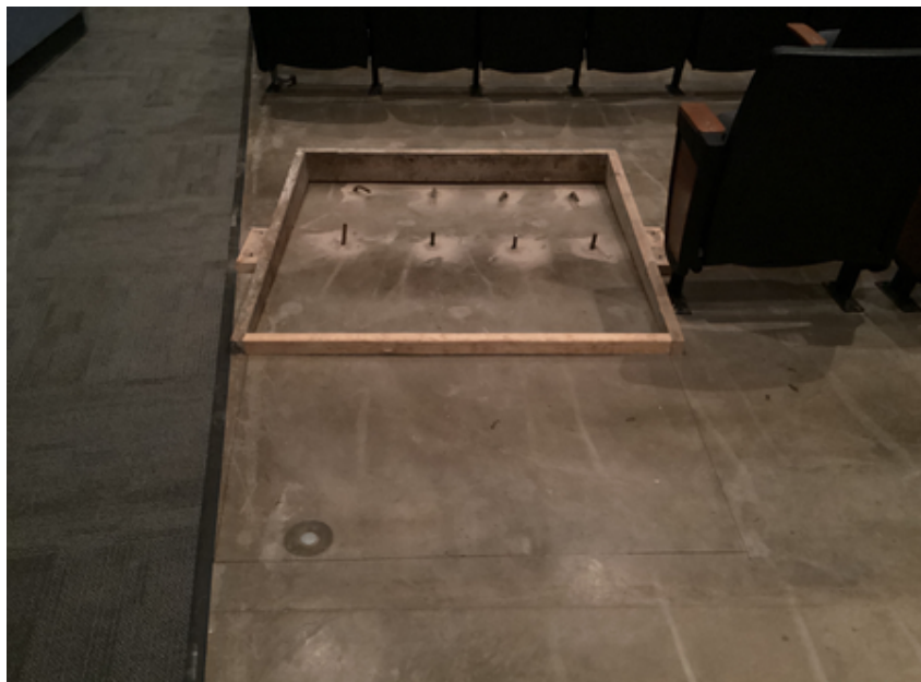
Forming ADA concrete platforms in Auditorium
