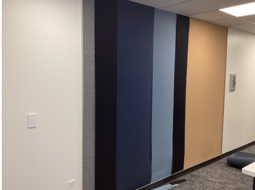
Wall coverings at Area C main entrance addition
