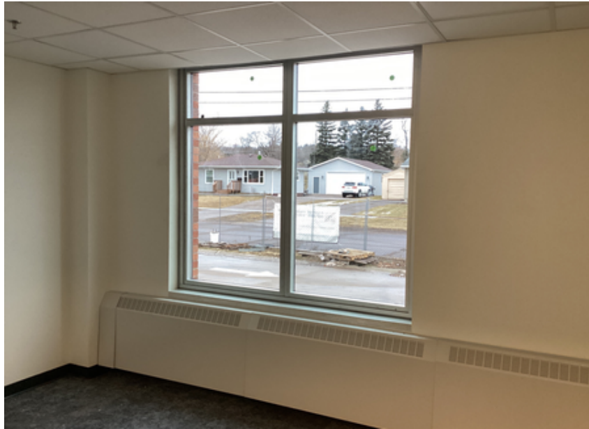
Window installation at Area C main entrance addition
