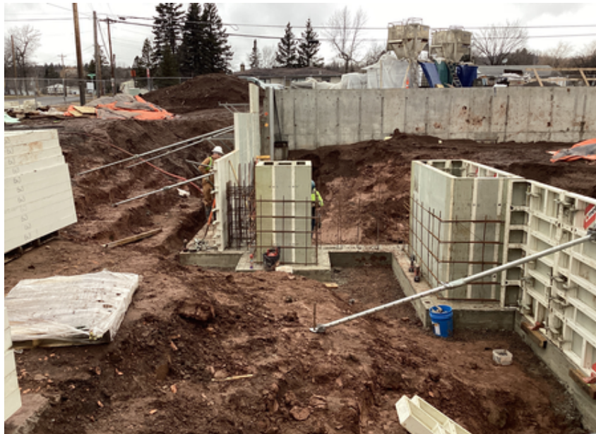
Last forms for foundations at Area B Music Suite
