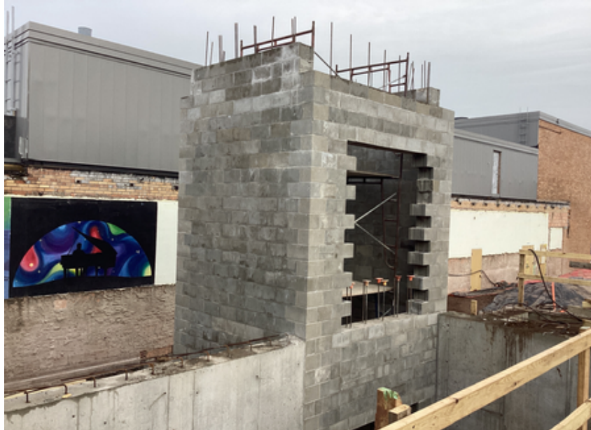
Elevator walls at Area B Music Suite
