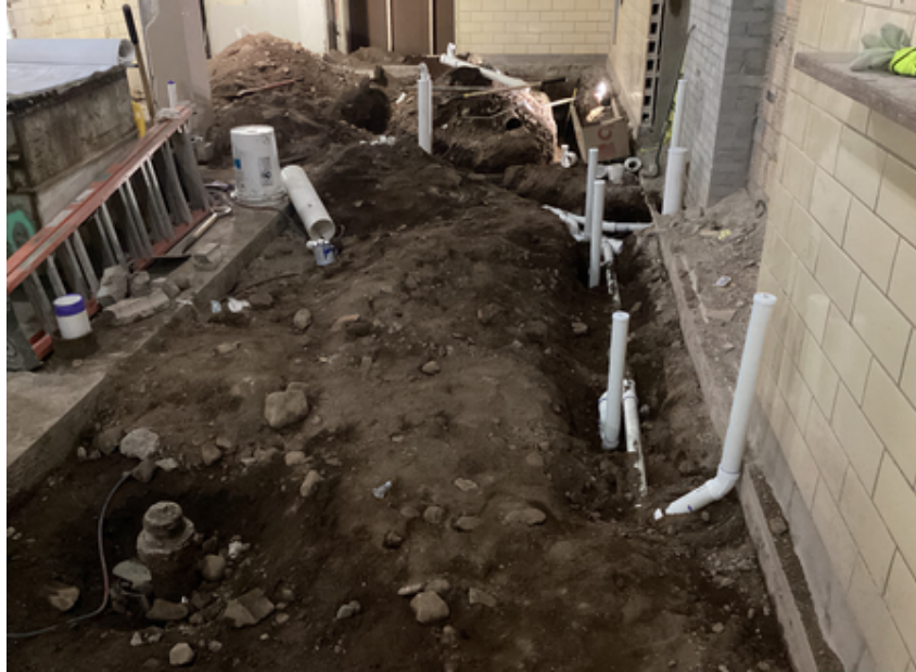
Underground plumbing in boys' locker room
