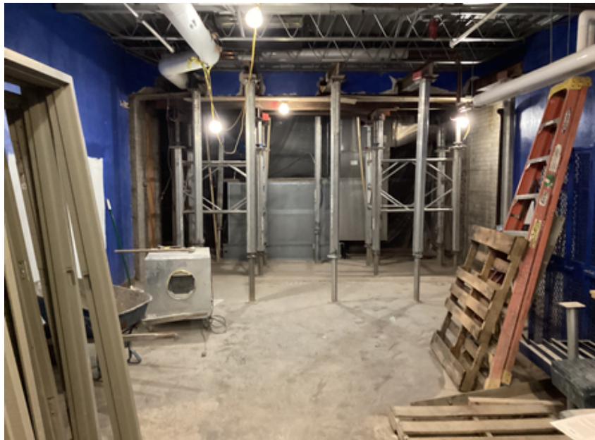
Demolition and structural shoring in boys' locker room
