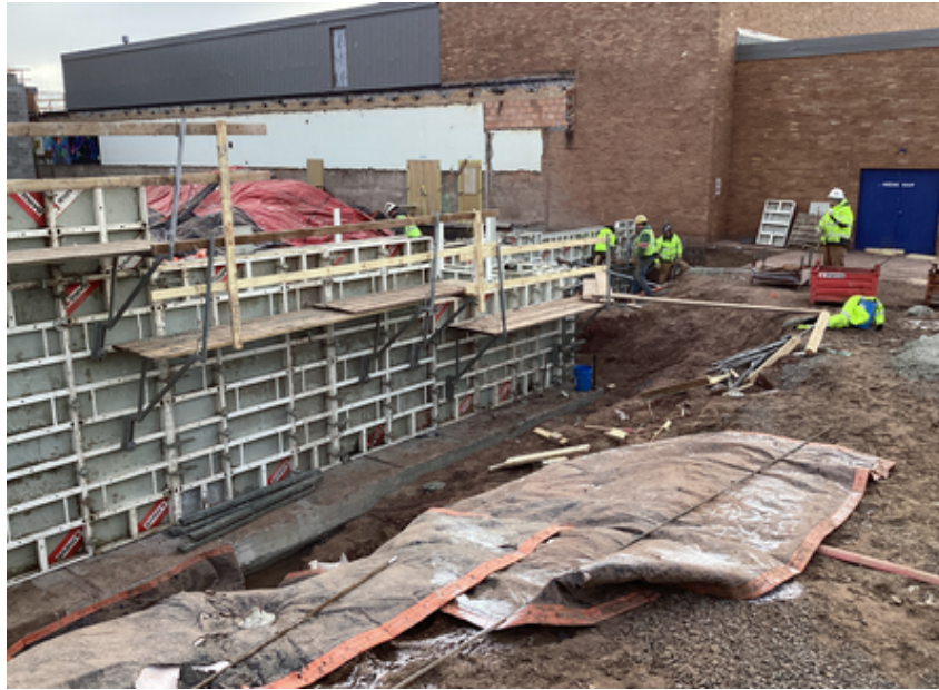
Last forms and pour for foundations at Area B Music Suite
