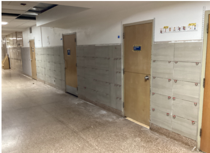
Corridor tile work main level
